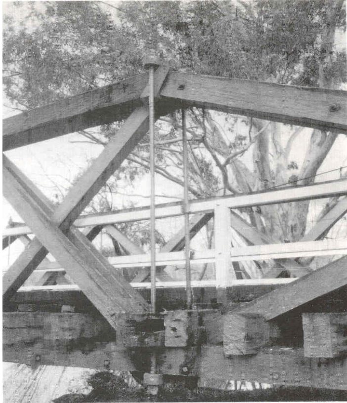
“Suspension roads in pairs either side of the timber.”
