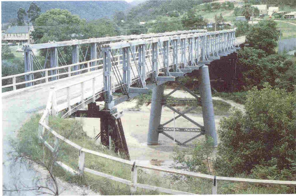
“De Burgh trusses over MacDonald River at St.Albans.”
