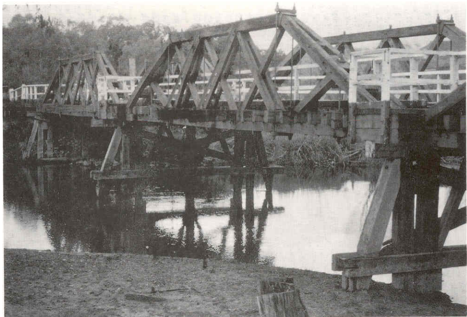
“Some diagonal members are single timbers, some are double timbers.”
