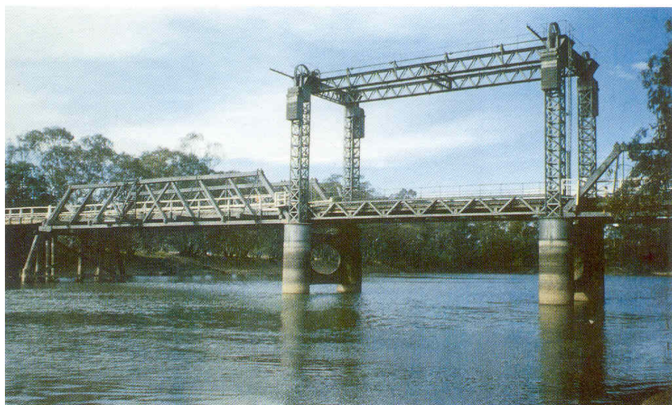
“Bridge over the Murray River at Swan Hill. 1896.”
