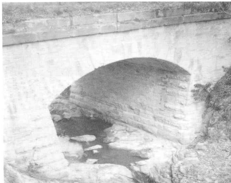
“Stone culvert at Towrang, near Goulburn, on Mitchell’s old route of the Hume Highway.”
