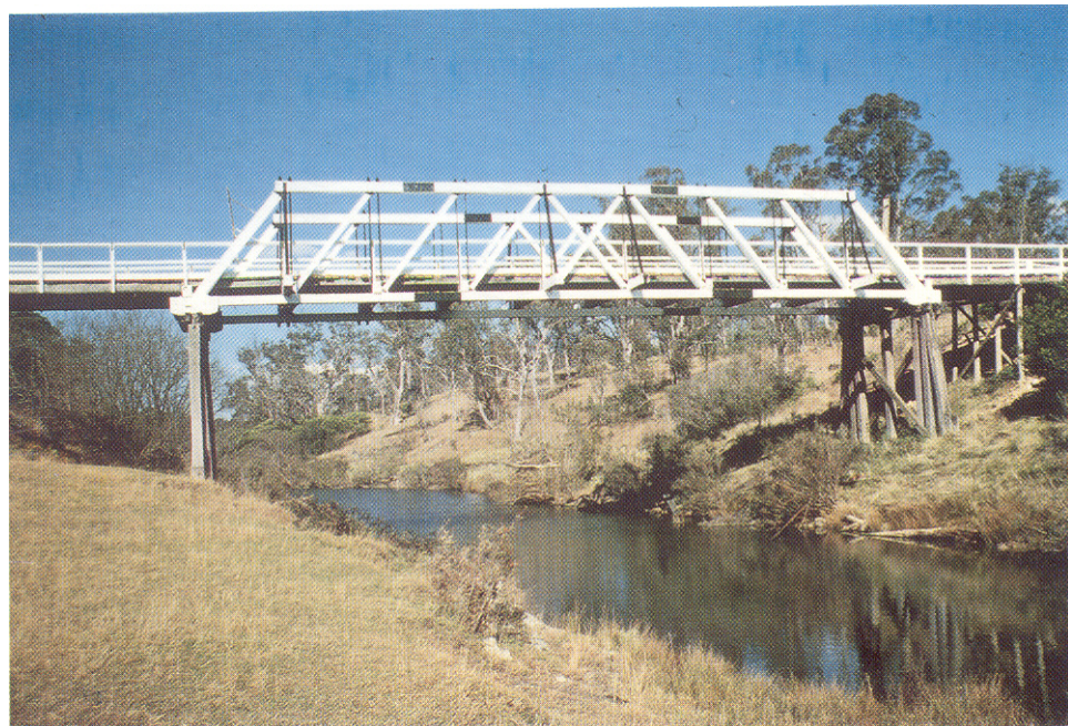
“Allan Truss over Molonglo River at Burbong.”
