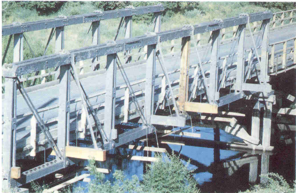
“Pratt type truss, designed by De Burgh, over Mulwaree Ponds, Goulburn.”
