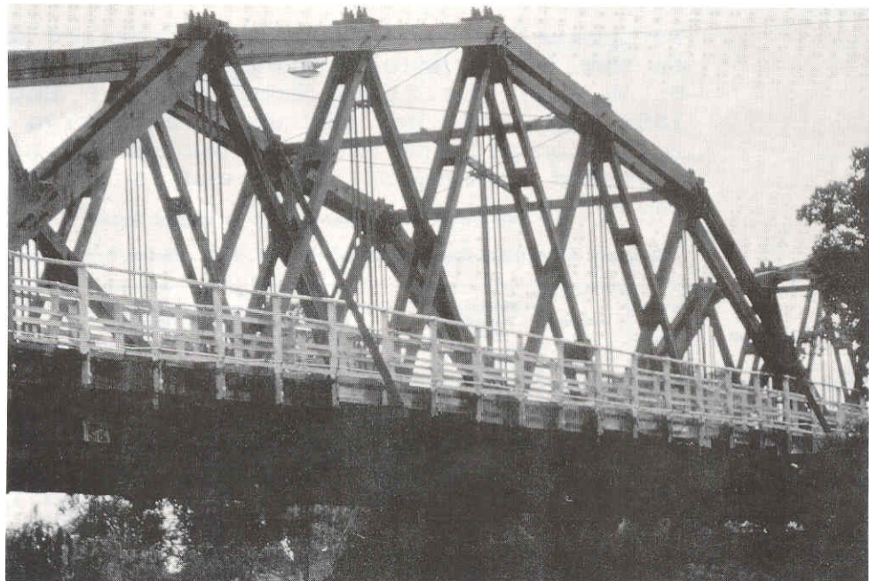
“ McDonald truss at Cowra showing principle features.”
