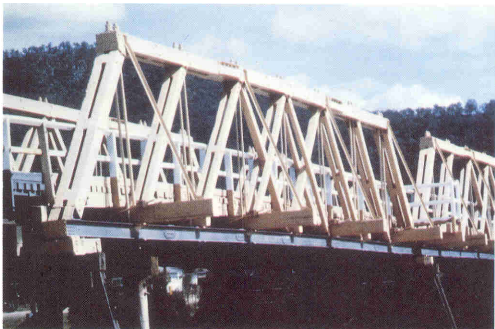
“Howe type truss, designed by Dare, over Wollombi Brook at Bulga.”
