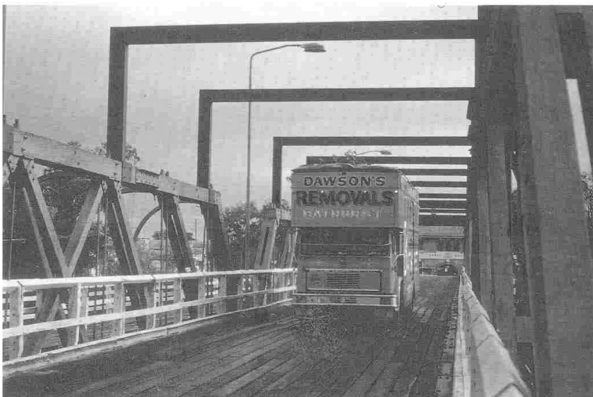
Figure 171: Portal Bracing used in the past to provide lateral restraint to bowing top chords.
