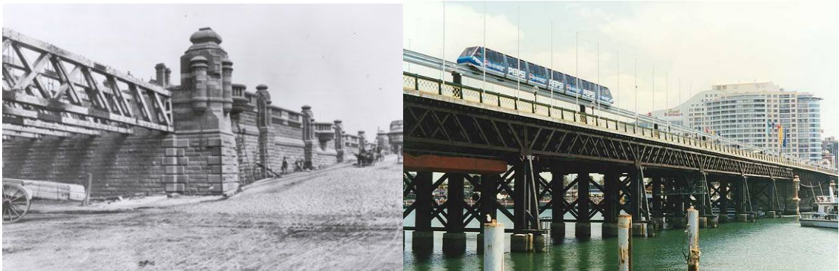
Figure 39: Allan Truss: Pyrmont Bridge with Six Allan Trusses Below the Deck on Each Span
