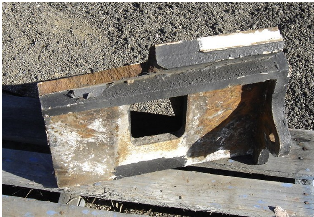
Figure 136: Brittle Fracture of Cast Iron Shoes in Allan Truss at Morpeth
