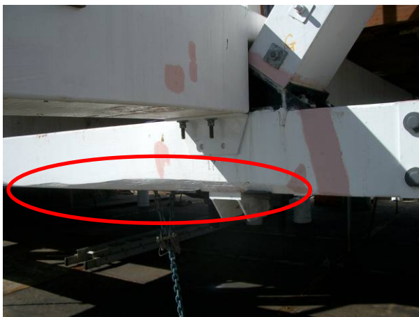
Figure 71: Rossi Bridge (Allan Truss) – bottom chord is not square due to removal of sapwood
