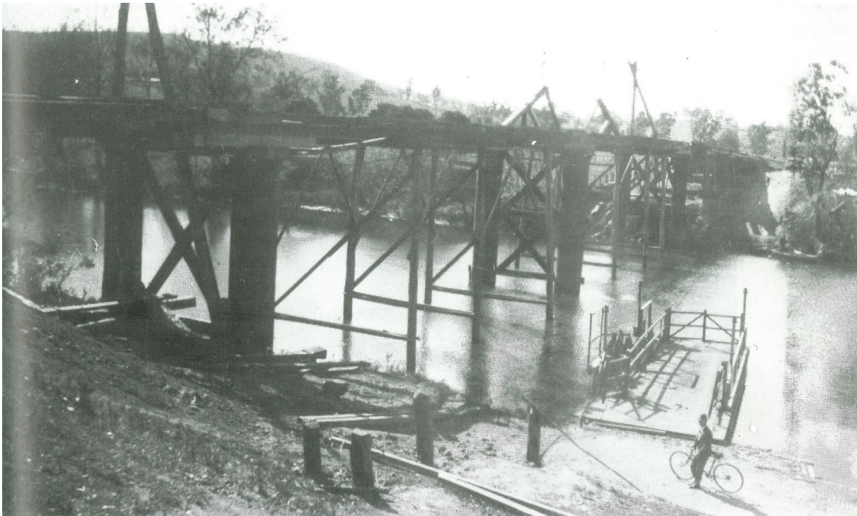
Figure 7: Construction of Old PWD truss at Clarence Town (R.L. Ford, Williams River, 1995, p 221)
