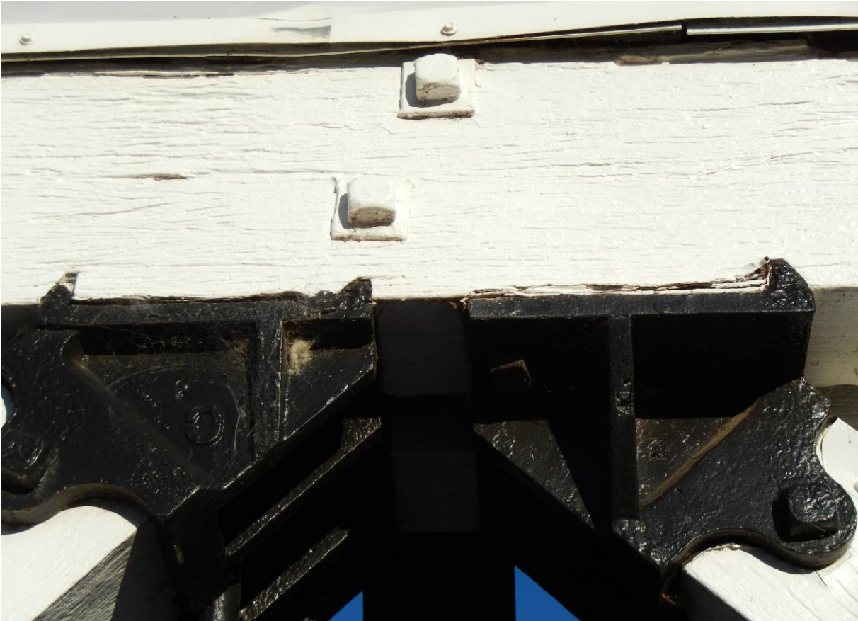
Figure 145: Deterioration at Top Chord Shoe in Dare Truss at Scabbing Flat
