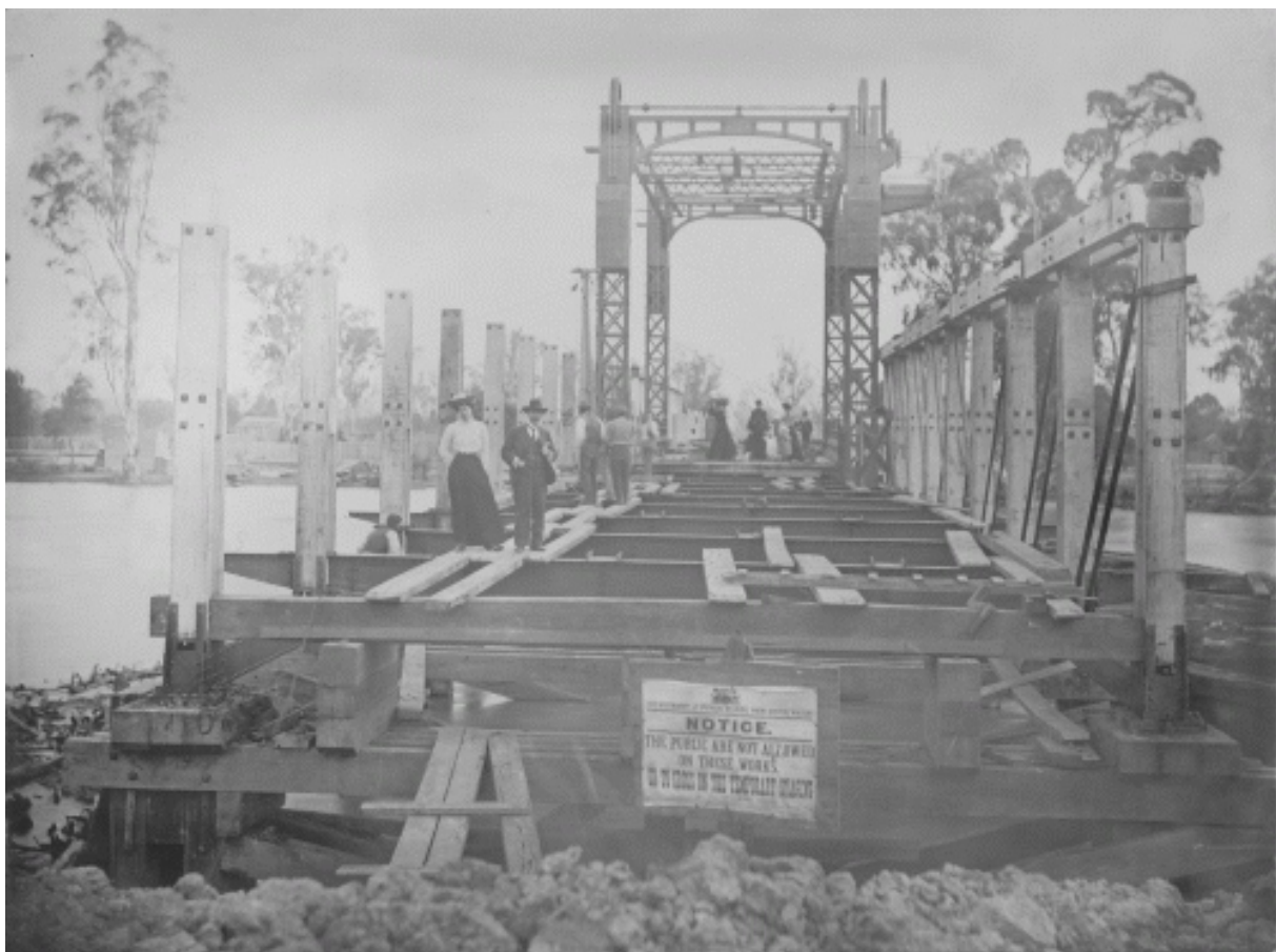
Figure 127: Construction of Barham Bridge with Vertical Struts Standing Unassisted.
