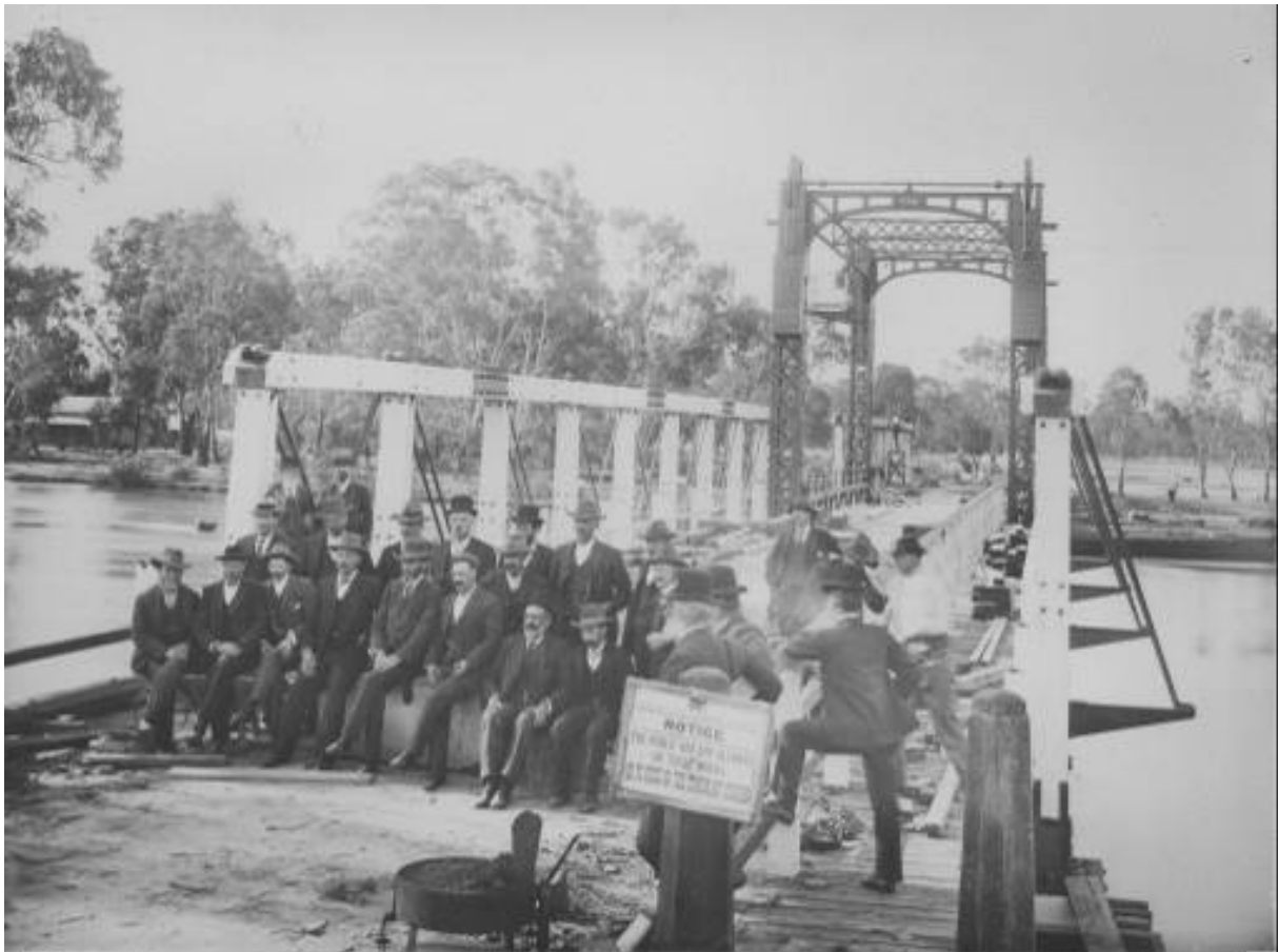
Figure 155: Construction of Barham Bridge (University of Melbourne Archives Image Collection)
