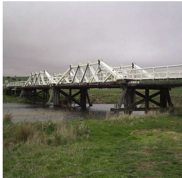
Figure 28: A “McDonald” Truss Bridge
