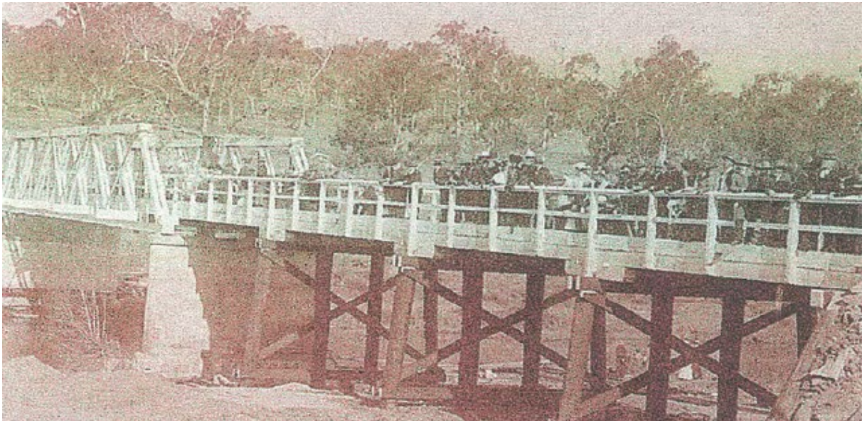
Figure 52: Opening of one of the first Dare Trusses: Bridge over the Macdonald River at Bendemeer
