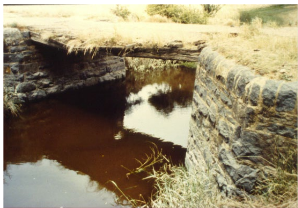
Figure 5: Early Bridges: A Turf Covered Bridge
