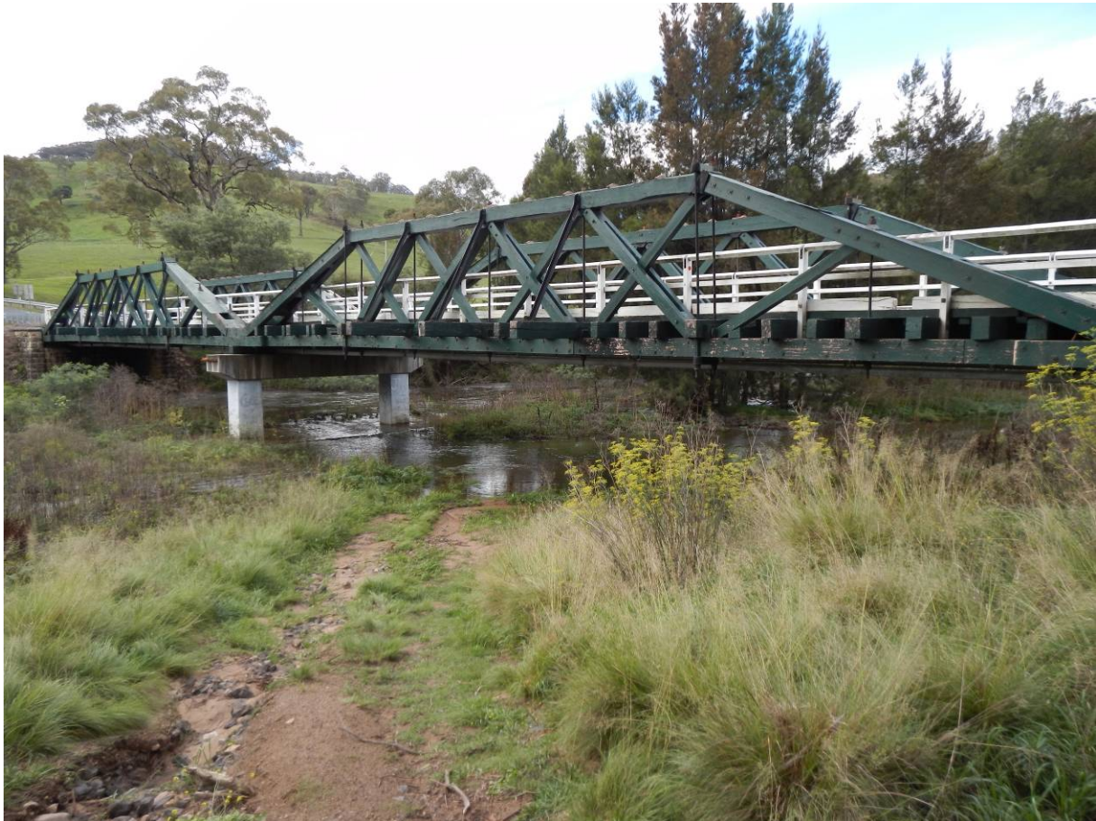
Figure 185: McKanes Bridge over the Cox's River near Lithgow
