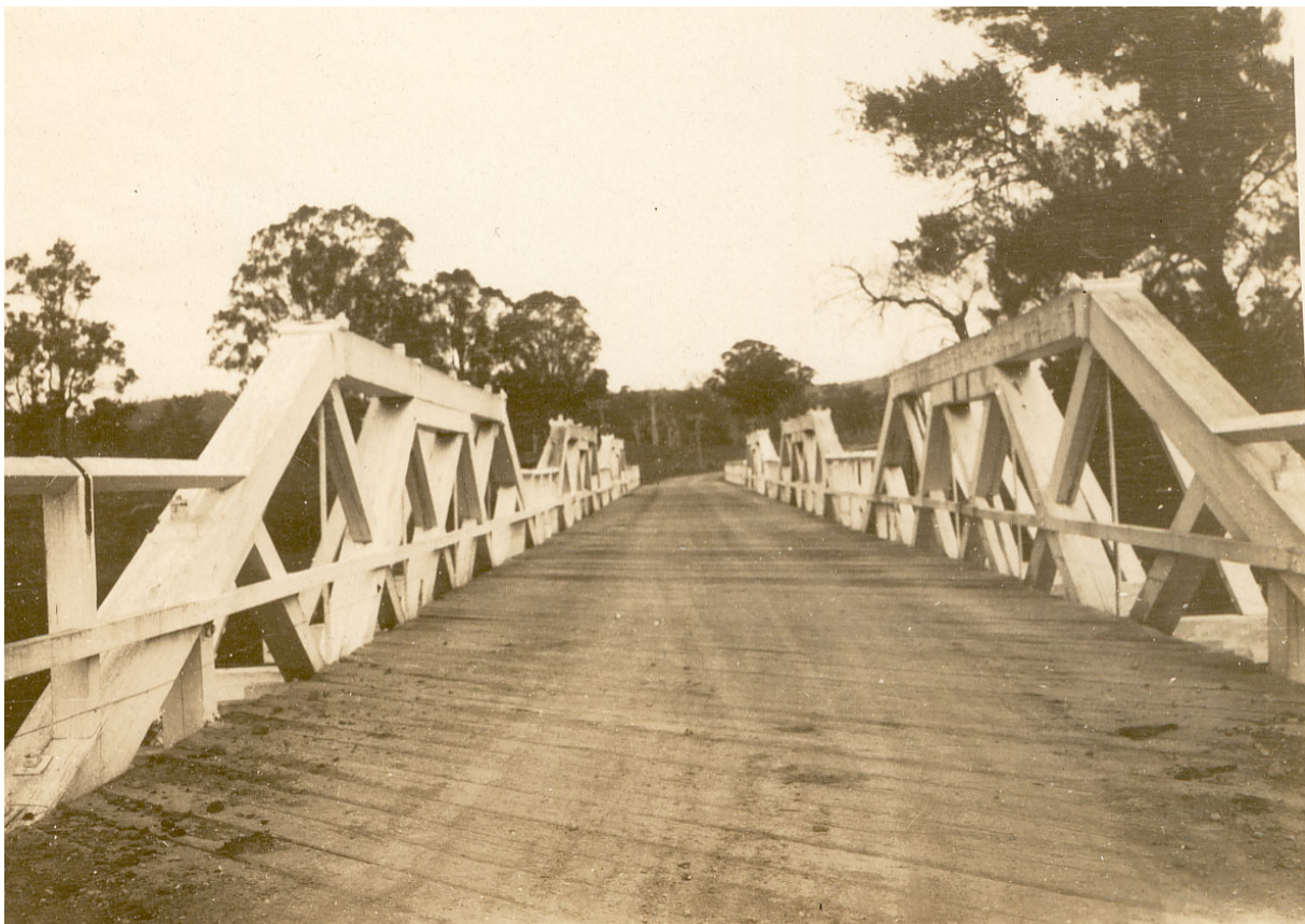
Figure 106: Photograph of Monkerai Old PWD trusses with Original Decking System
