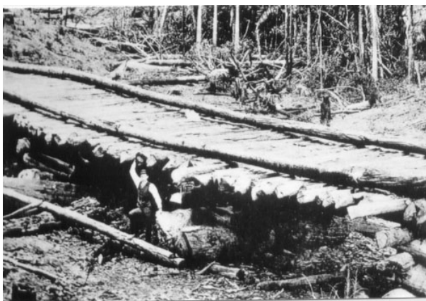
Figure 4: Early Bridges: A Corduroy Bridge
