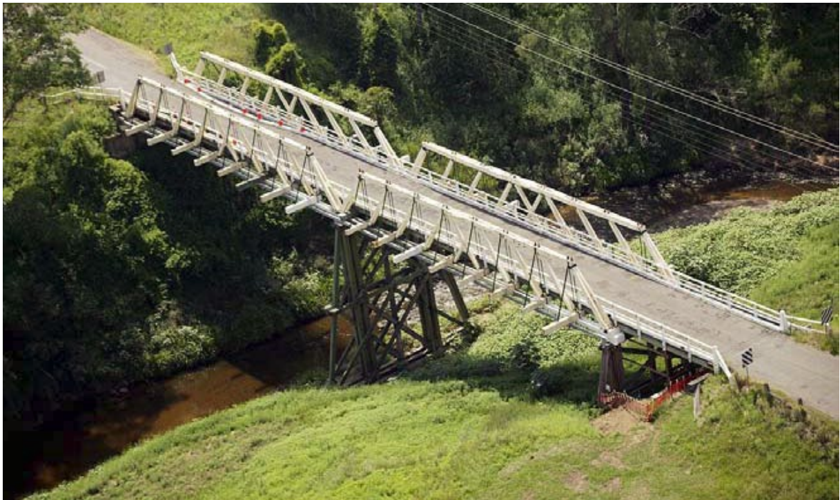
Figure 40: Allan Truss: Vacy Bridge over the Patterson River near Dungog
