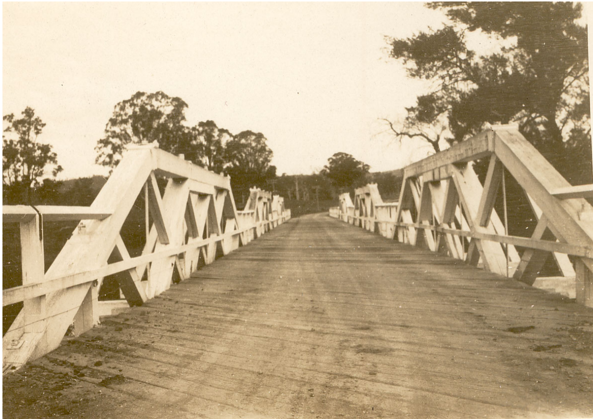
Figure 197: Monkerai Bridge over the Karuah River, as constructed in 1882
