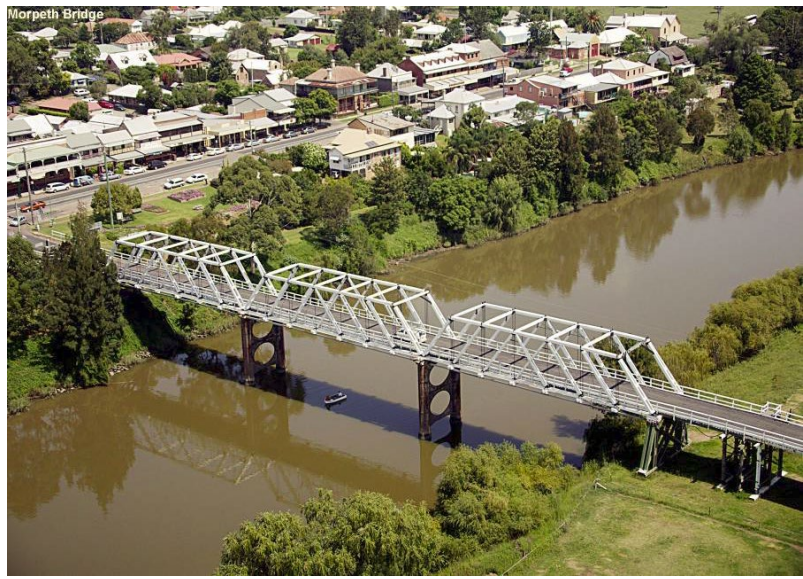
Figure 35: An “Allan” Truss Bridge
