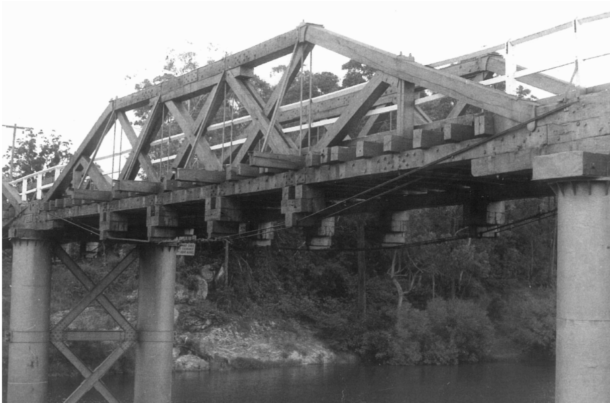
Figure 178: Clarence Town Bridge with Under-trussing (photograph taken in 1974)
