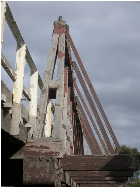
Figure 126: Lateral Buckling of Top Chord in Allan Trusses (Thornes Bridge and Euminbah)
