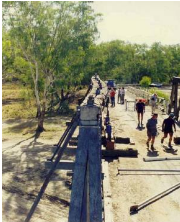
Figure 126: Lateral Buckling of Top Chord in Allan Trusses (Thornes Bridge and Euminbah)
