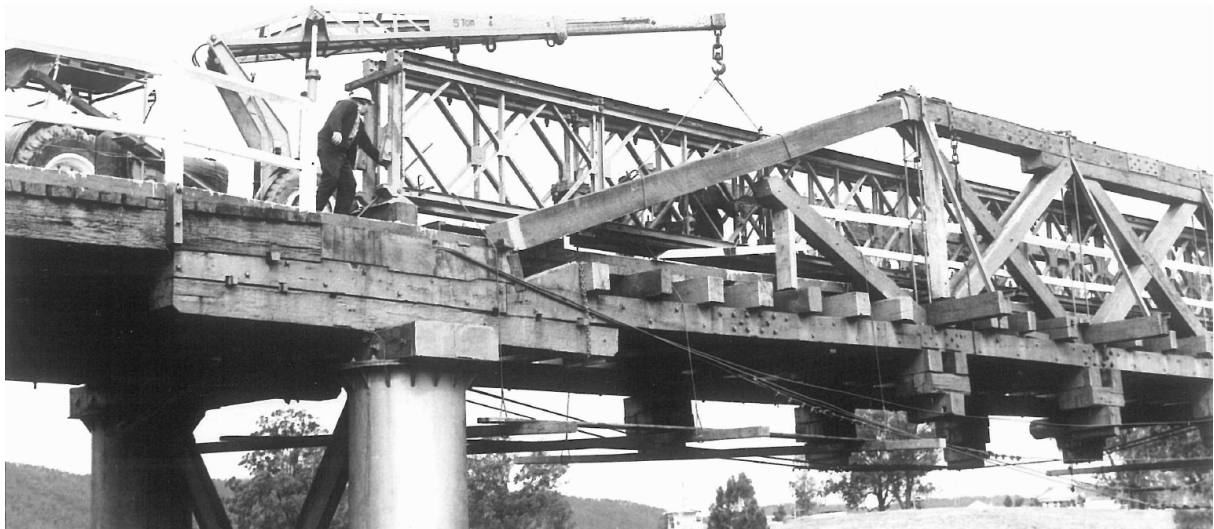
Figure 179: Replacement of Principal in 1975 using a Bailey Bridge (note under-trussing present too)
