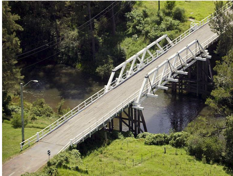
Figure 51: A “Dare” Truss Bridge
