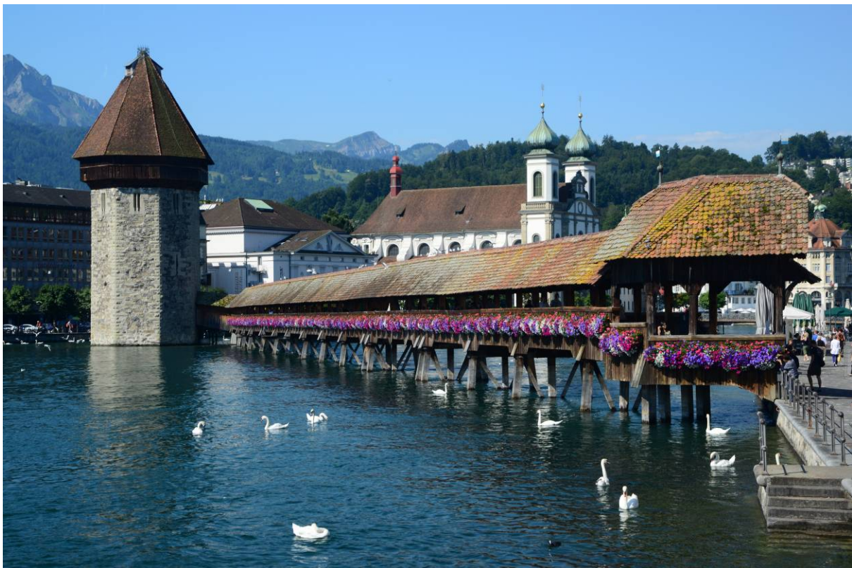
Figure 73: Photograph taken in 2012 showing the Kapellbrücke in Luzern, built in 1333
