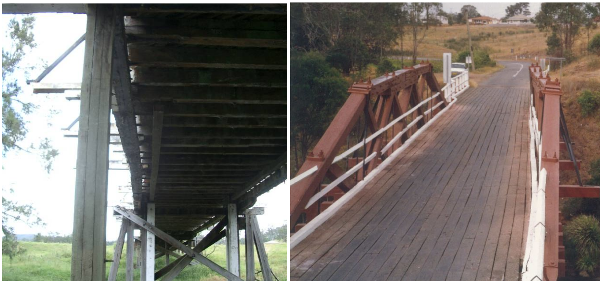
Figure 92: Left: Monkerai Bridge Bottom Chord, Right: Clarence Town Bridge Top Chord
