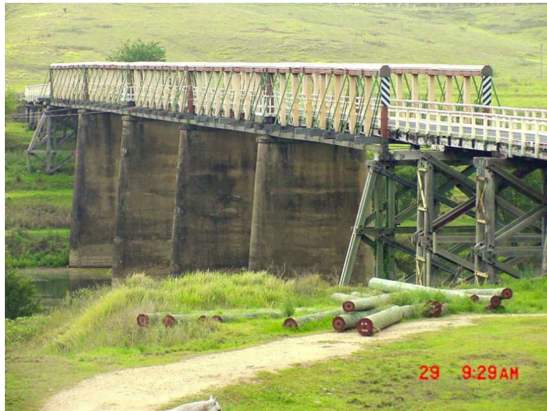
Figure 43: A “de Burgh” Truss Bridge
