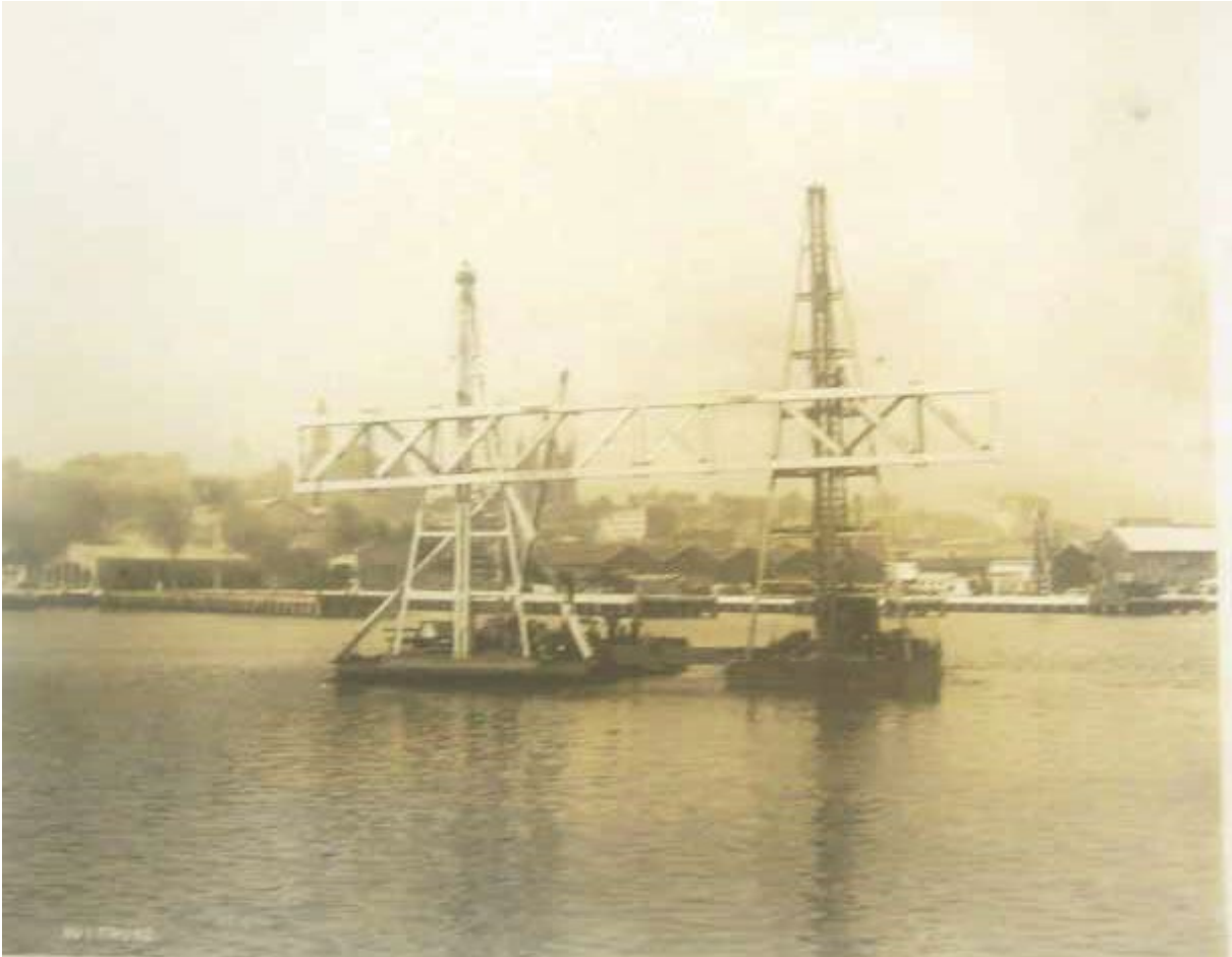
Figure 8: Construction of Allan Truss at Pymont (Pymont Bridge Conservation Management Plan)
