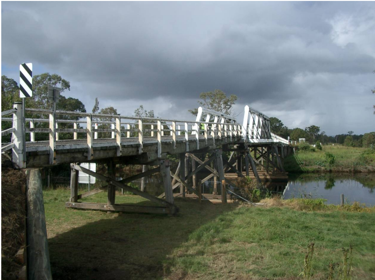
Figure 164: Briner Bridge over the Upper Coldstream River
