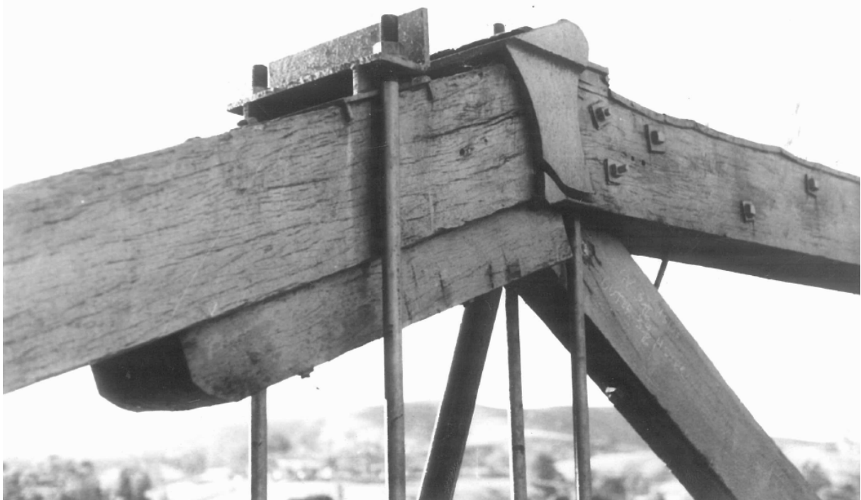
Figure 179: Replacement of Principal in 1975 using a Bailey Bridge (note under-trussing present too)
