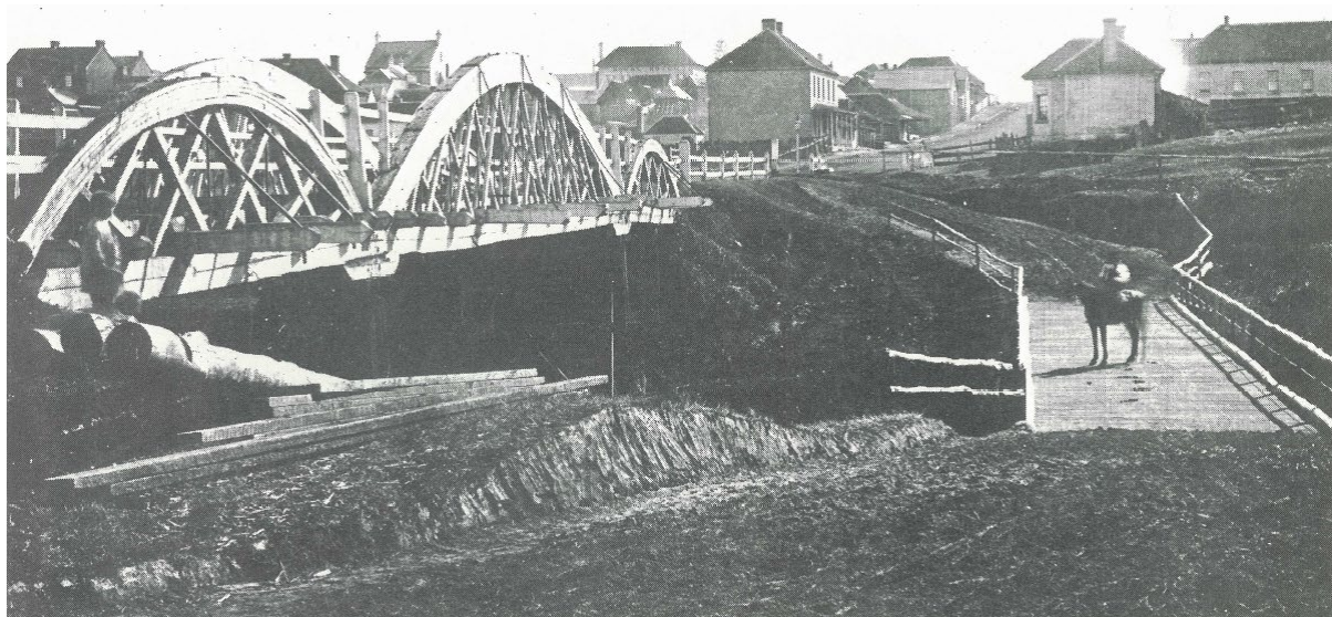
Figure 6: A Laminated Timber Arch Bridge over South Creek at Windsor
