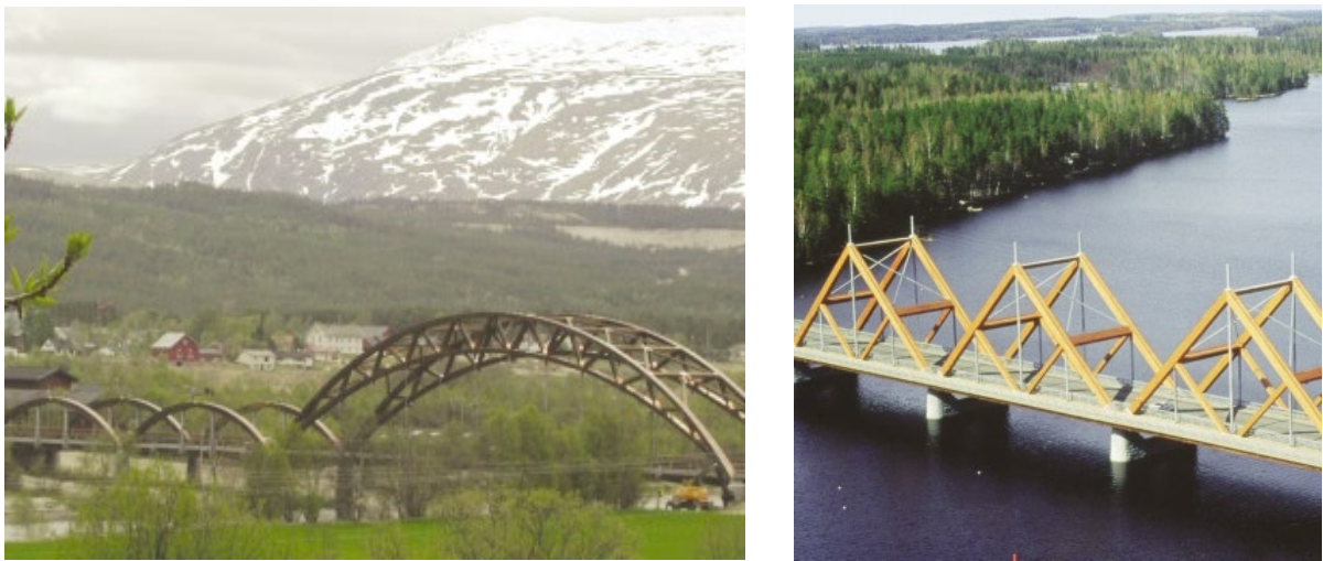
Figure 80: Norwegian Timber Bridges (photos from Nordic Innovation, 2002)
