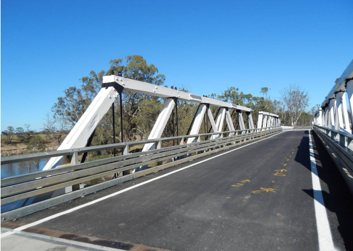
Figure 153: Barriers different darker colour from truss, thereby letting truss draw the attention
