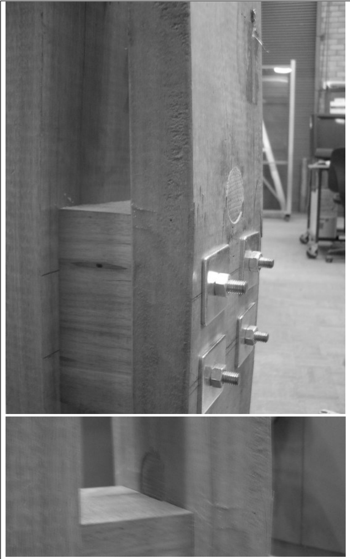
Figure A.13: Photographs of failure locations for Assembly 11A10A
