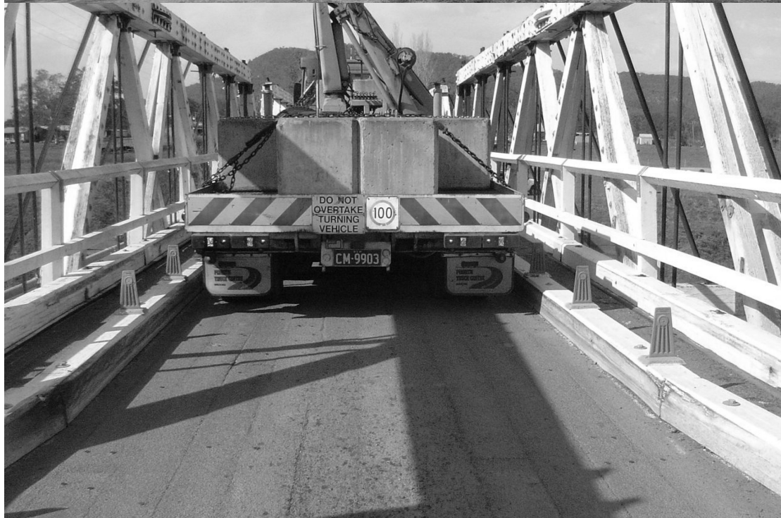
Figure 1.4: Load Testing and Strain Gauging of Vacy Bridge, Hunter Region 13
