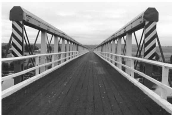
Figure 2.2: Photograph and Microstran Model of Tabulam Bridge – DeBurgh Truss
