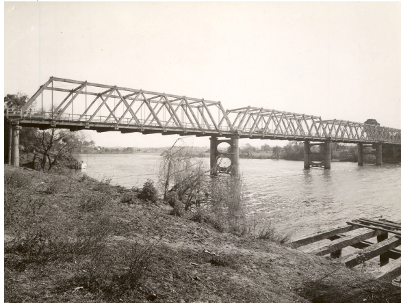
Fig 9. Macleay River Bridge at Kempsey, NSW (built 1900 replaced 1959) featured four 153ft timber spans (RTA Photo Archive).
