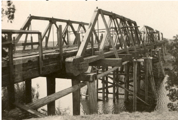
Fig 14. Bushy Park Bridge over the Avon River, west of Briagalong, Victoria under construction in 1926 (VicRoads Archives).
