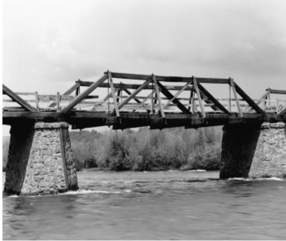
Figure 5: Squirrel Bridge, Fremont County, Idaho, USA (Idaho Department of Transport)
