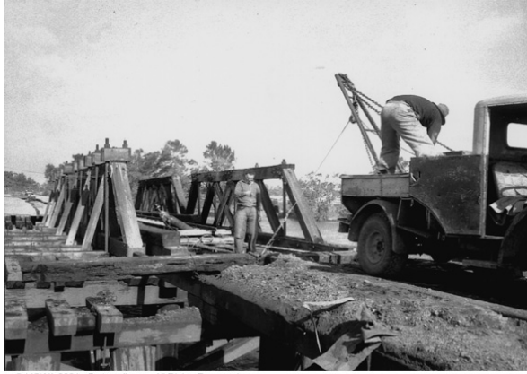
Fig 16. Workers demolishing the Belmont Railway Bridge, East Perth in 1957 (Batty Library, WA, Call # BA1218/13). Note the principals and diagonals are solid, heavy members.
