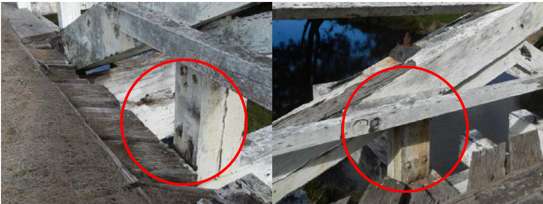
Figure 3-11: Photo showing vertical props consisting of two timbers bolted.
