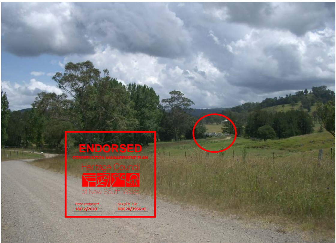
Figure 1-6: View 2 of Bridge approaching from the north 250m from bridge
