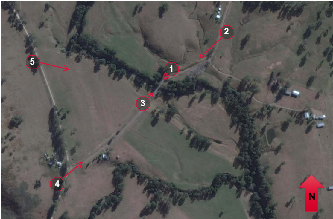
Figure 1-4: Aerial View of Bridge with locations from which views are seen.
