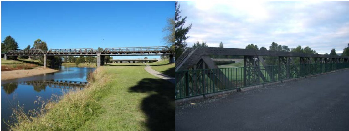
Figure 2-23: Denison Bridge Bathurst, Macquarie River today.
