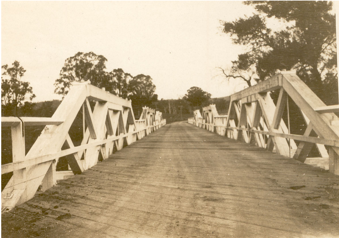
Figure 2-35: First Available undated photograph of Monkerai Bridge.
