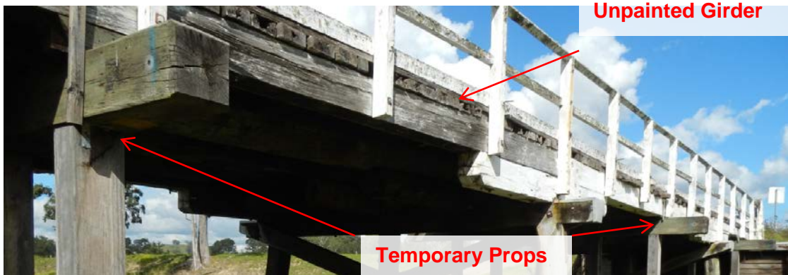
Figure 3-30: Photograph showing unpainted girder and temporary props.
