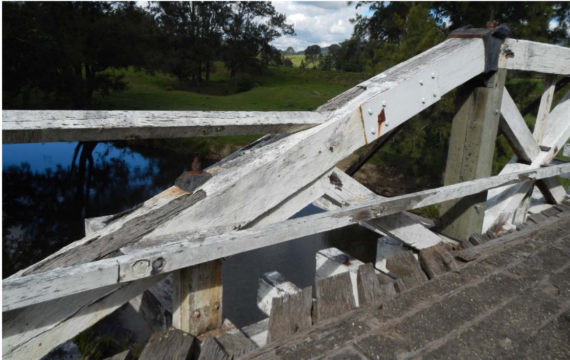
Figure 3-41: Photograph showing edge of deck from on top of truss span.
