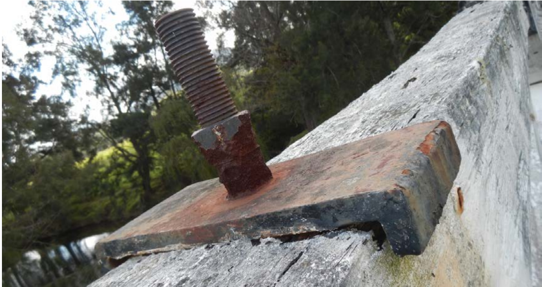
Figure 3-21: Photo of wrought iron washer plate at top of tension rod.
