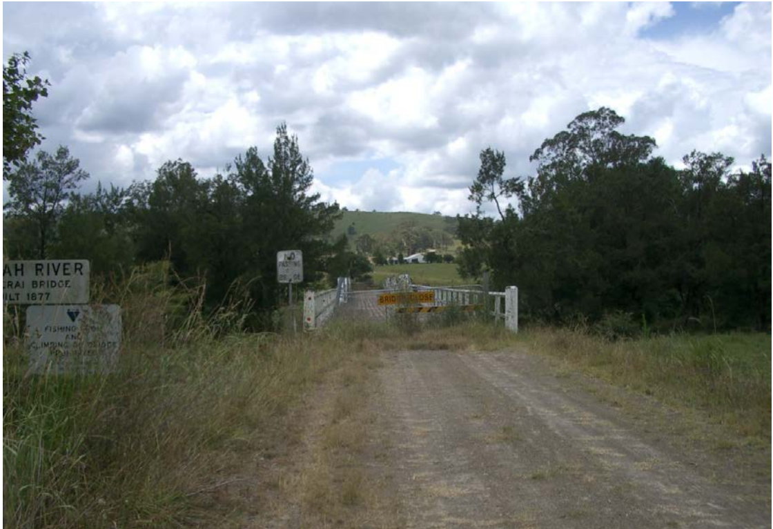
Figure 1-7: View 3 of Bridge approaching from the south close to bridge.
