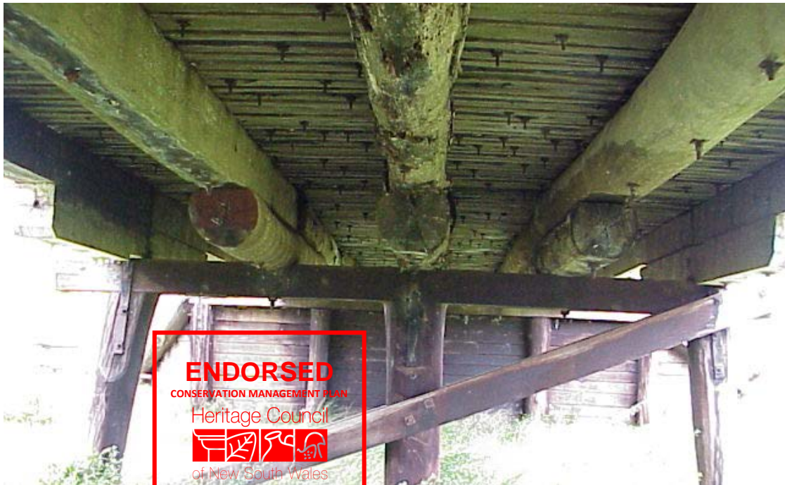
Figure 3-34: Photograph of bolts viewed beneath approach spans.
