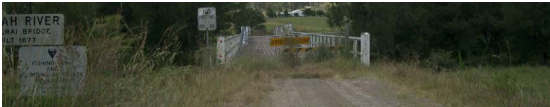
Figure 3-42: Photograph showing end posts which have been added.
