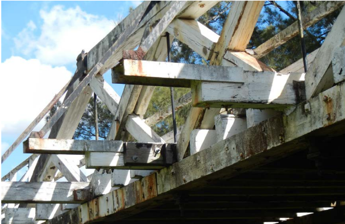
Figure 3-25: Photo of current metal sway braces and metal CG extensions.
