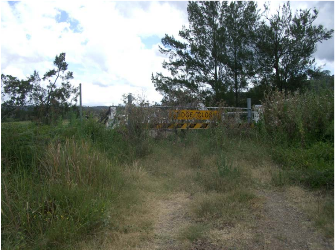
Figure 1-5: View 1 of Bridge approaching from the north close to bridge.
