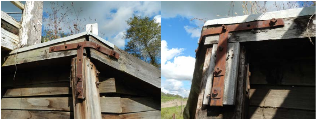
Figure 3-49: Metal straps on Abutment A possibly original fabric.
