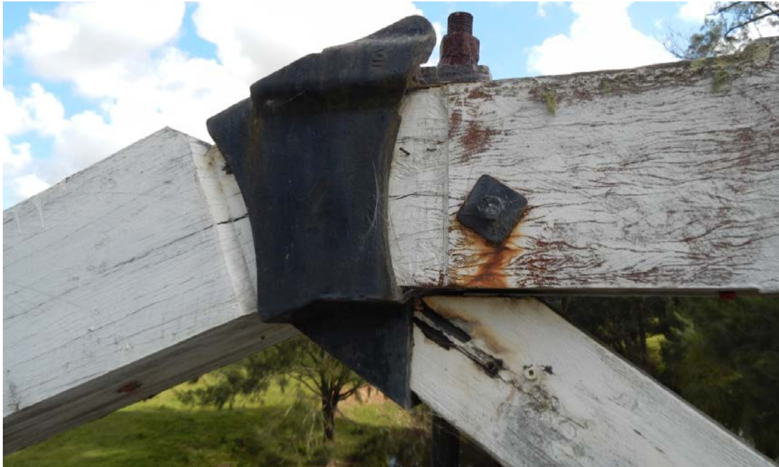
Figure 3-15: Photos of typical top chord cast iron shoe.
