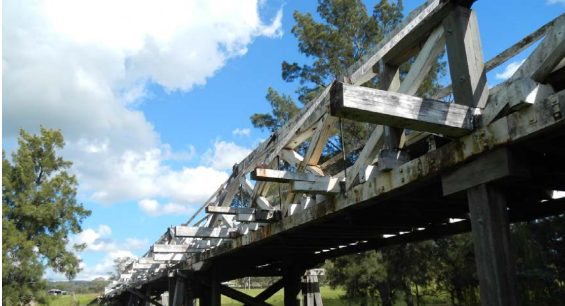
Figure 3-24: Photo of current metal sway braces and metal CG extensions.
