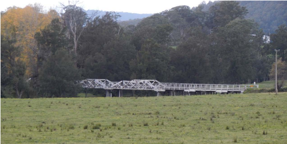
Figure 1-2: Photograph of Monkerai Bridge in its setting from distance.
