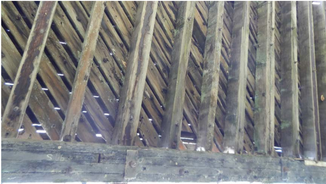
Figure 3-38: Photograph showing view of deck from beneath truss span.
