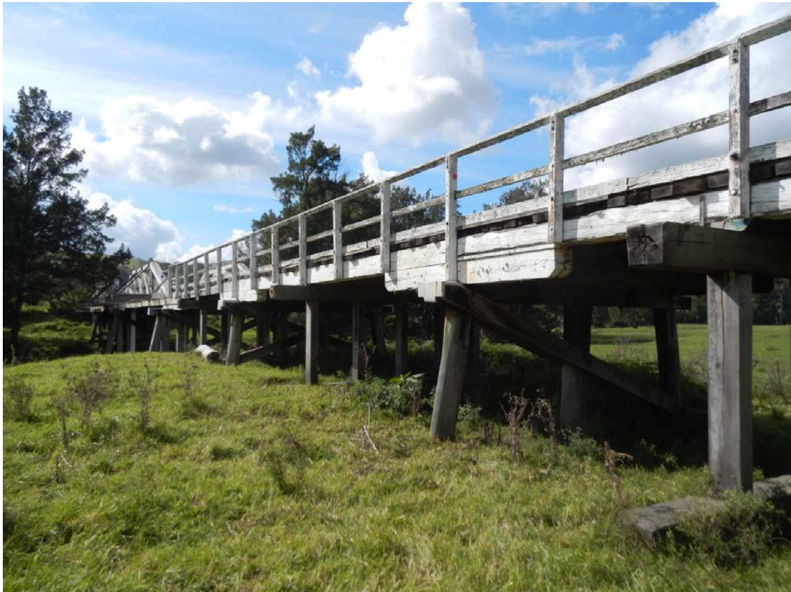
Figure 3-32: Photograph showing current detailing of approach spans.
