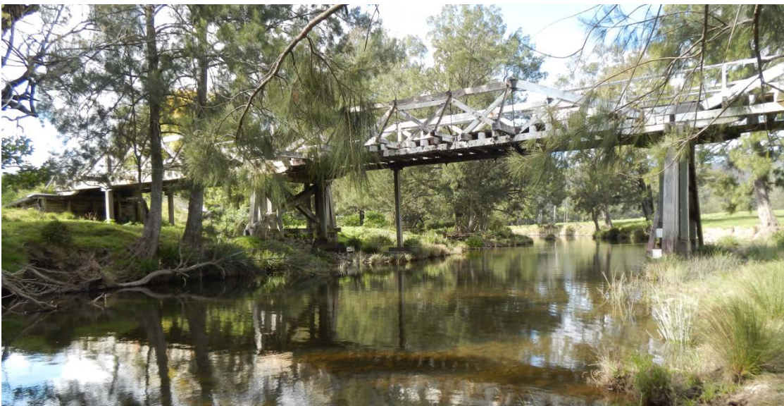
Figure 1-3: Photograph of Monkerai Bridge in its setting from close.
