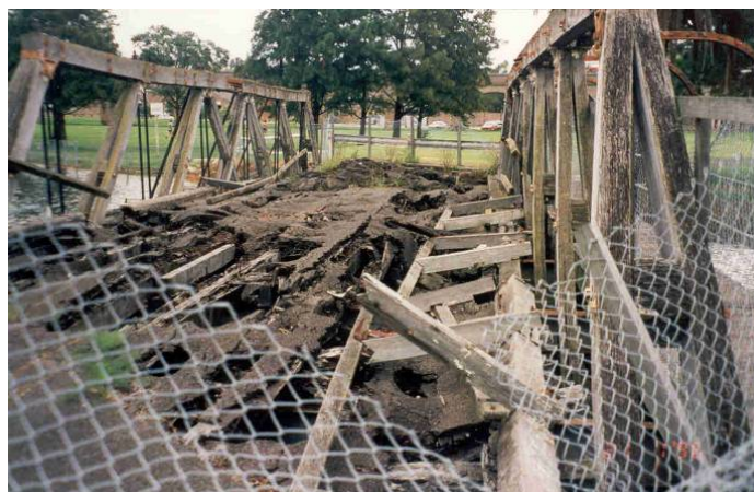
Figure 6.1 Johnston's Creek Bridge, Glebe (source: J. McPhail)
