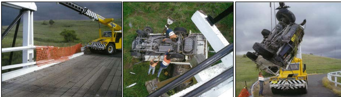
Figure 6.2 Photographs of vehicle recovery after crash on a de Burgh truss in Hunter Region (source: RMS)
