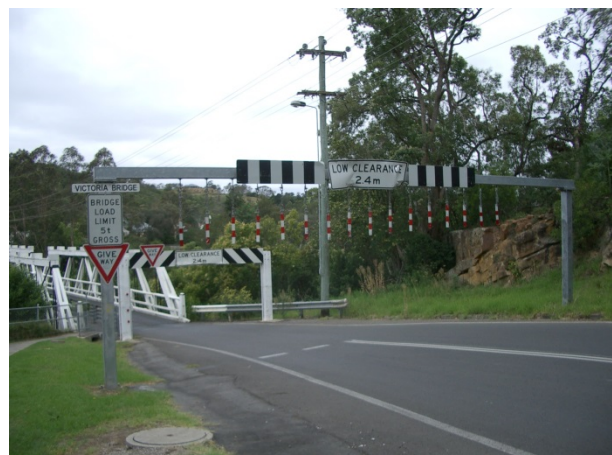
Figure 7.1 Load Limit at Victoria Bridge (source: author)
