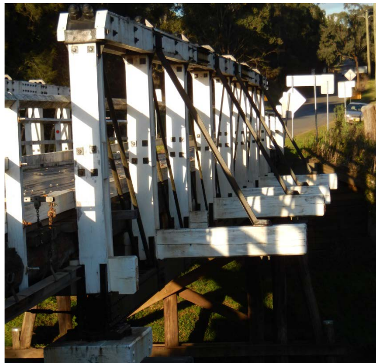
Figure 4.12 Photograph of Sway Braces (Source: Author, 2013)
