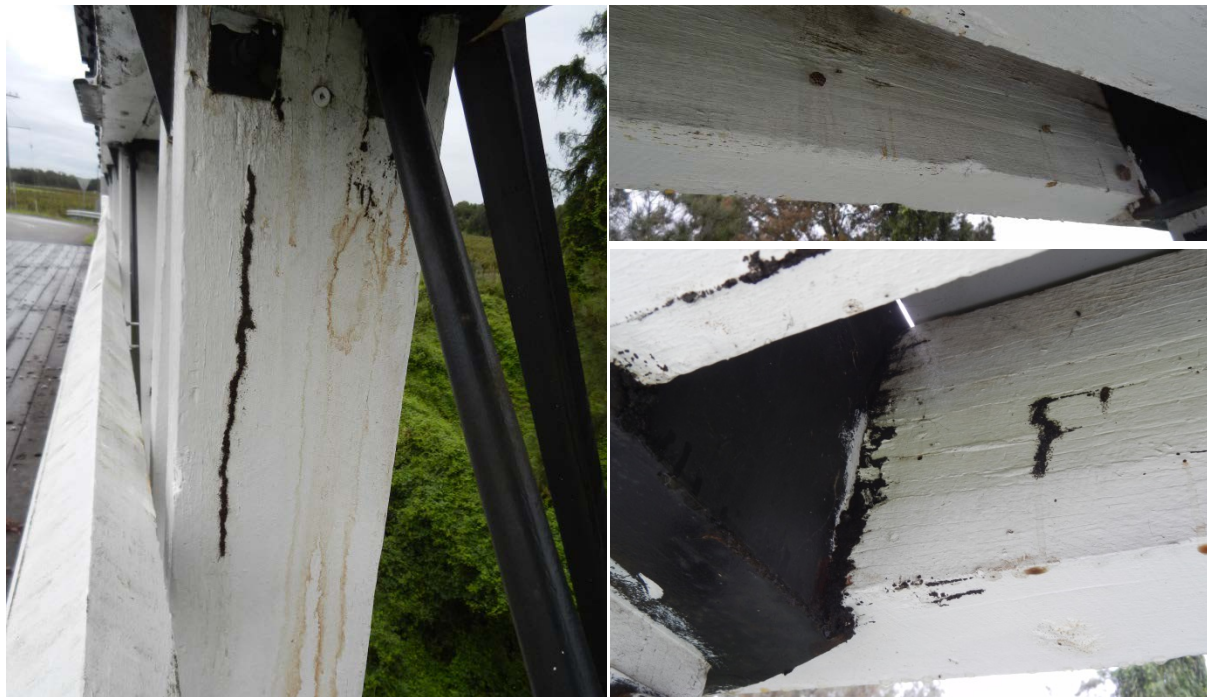
Figure 7.5 Photographs of termites and wasps in top chords and verticals (source: Author, March 2017)
