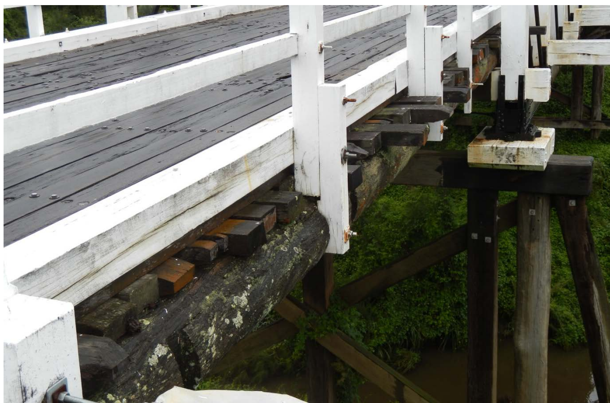
Figure 7.12 Photograph of current approach span configuration (source: author, March 2017)
