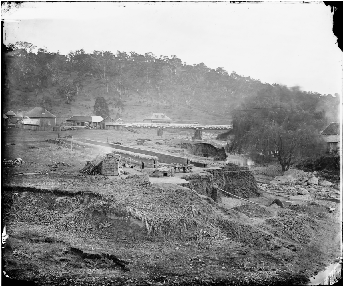
Figure 3.6 First Timber Truss Bridge in NSW constructed over the Belubula River at Carcoar in 1855/56 (Source: American & Australasian Photographic Company, Brick-making on the banks of the river at Carcoar, looking south, from the collections of the State Library of New South Wales, date of work approx. 1870 – 1875)
