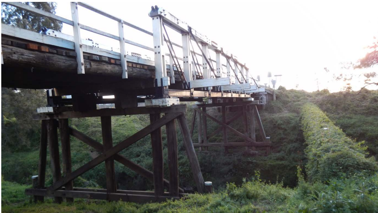
Figure 4.18 Photograph showing configuration of current piers and abutments (source: author)
