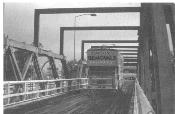
Figure 7.11 Overhead portal bracing (source: RMS)
