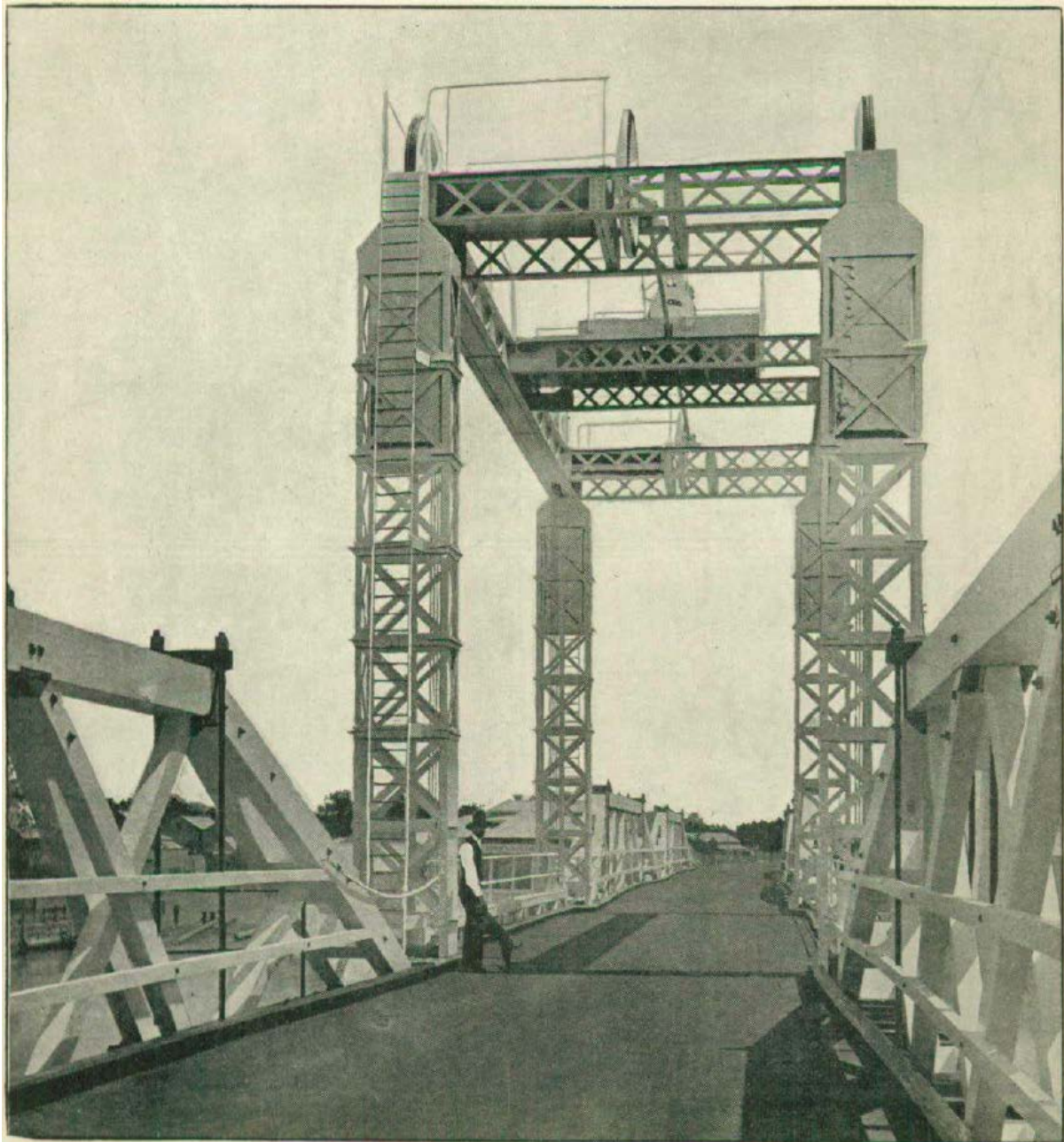
Figure 4.15 Original Timber Deck on Timber Truss Bridge over Darling River at Wentworth in 1894
