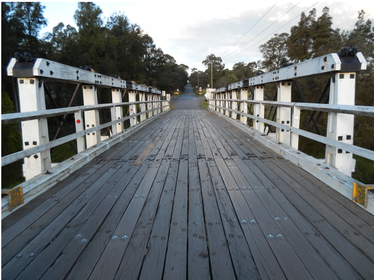
Figure 2.3 Photograph of Gillies Bridge (source: author, August 2013)
