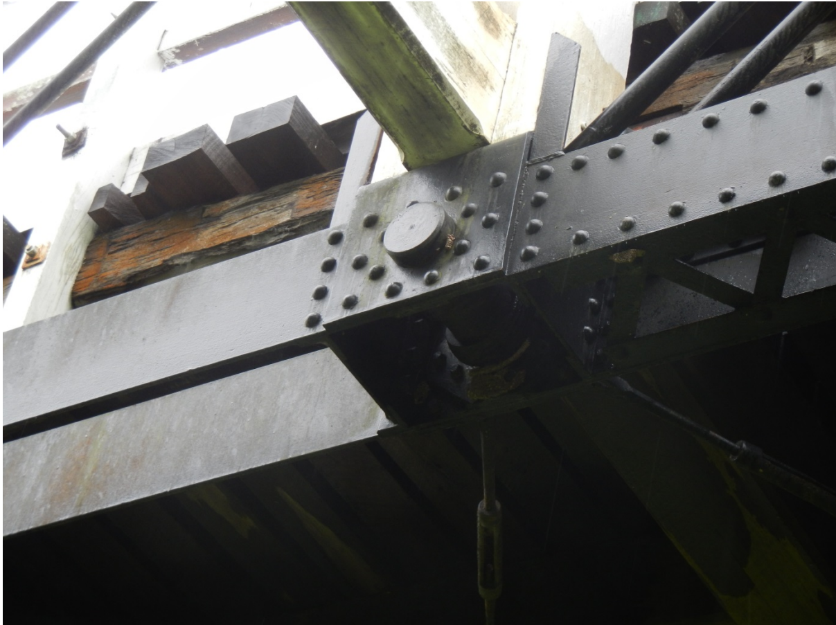
Figure 4.9: Photograph showing various bottom chord details at panel point (source: author 2017)
