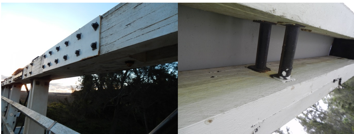
Figure 7.7 Photographs non-original details including splice on left and spools on right (source: Author)
