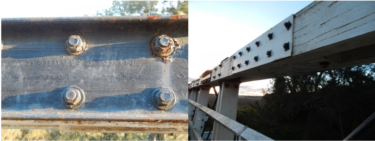
Figure 4.3: Left: Original Splice Plate with Foundry Mark; Right: Introduced splice plate (source: author 2013)
