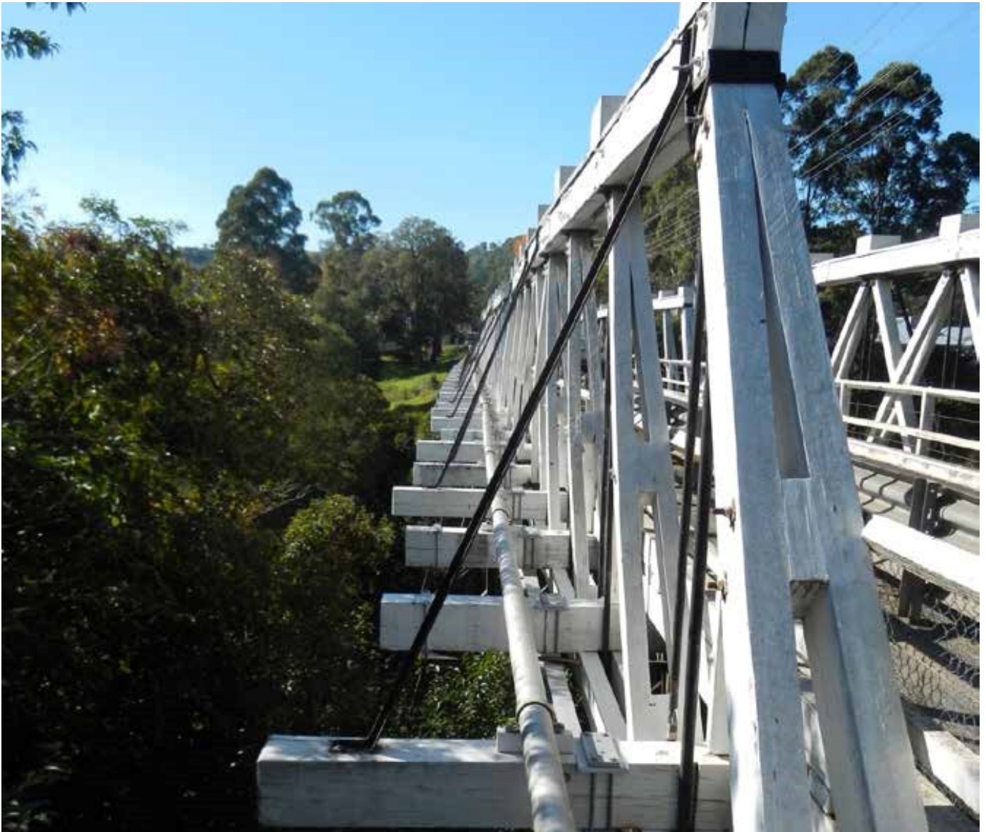
Figure 2-69: Photographs of upstream sway braces at Victoria Bridge
