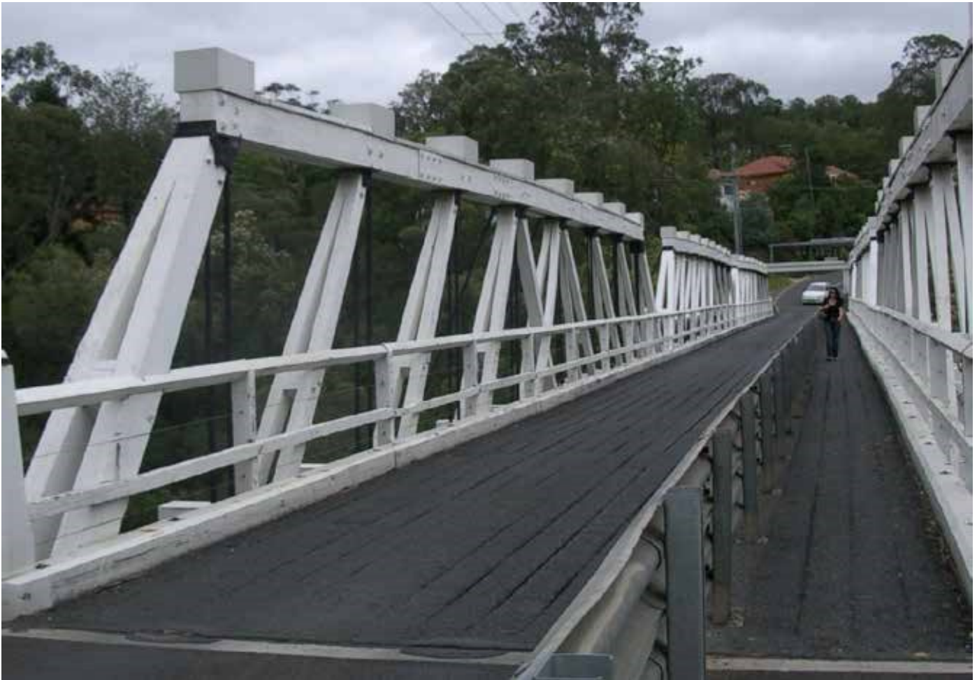
Figure 2-80: Photo of existing longitudinal sheeting viewed from above
