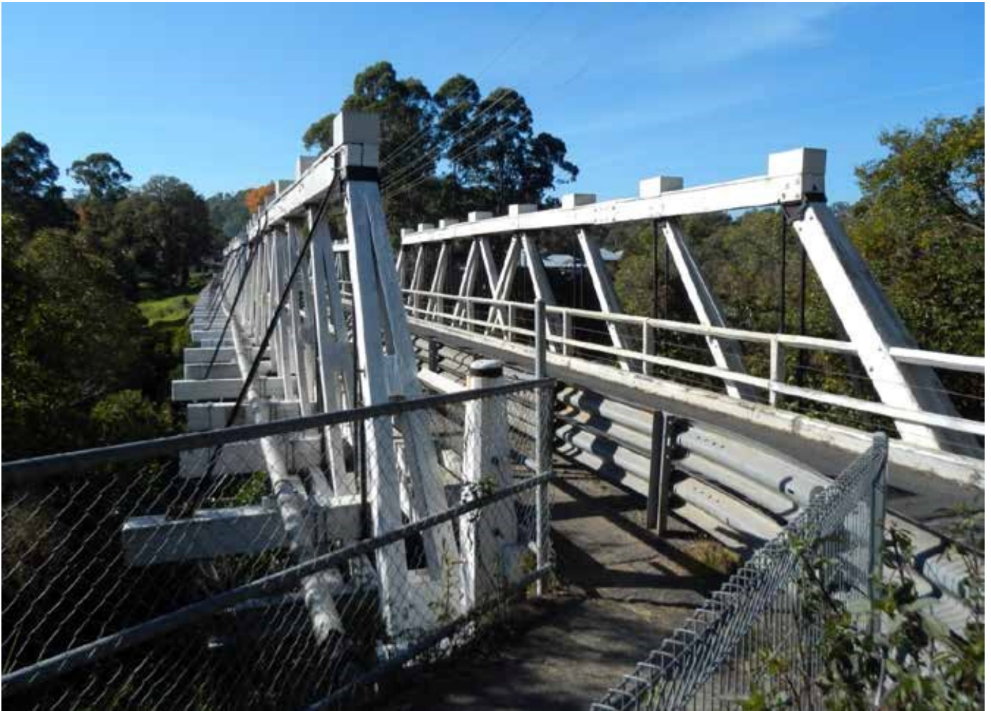
Figure 2-74: Photo showing existing non-original long cross girders
