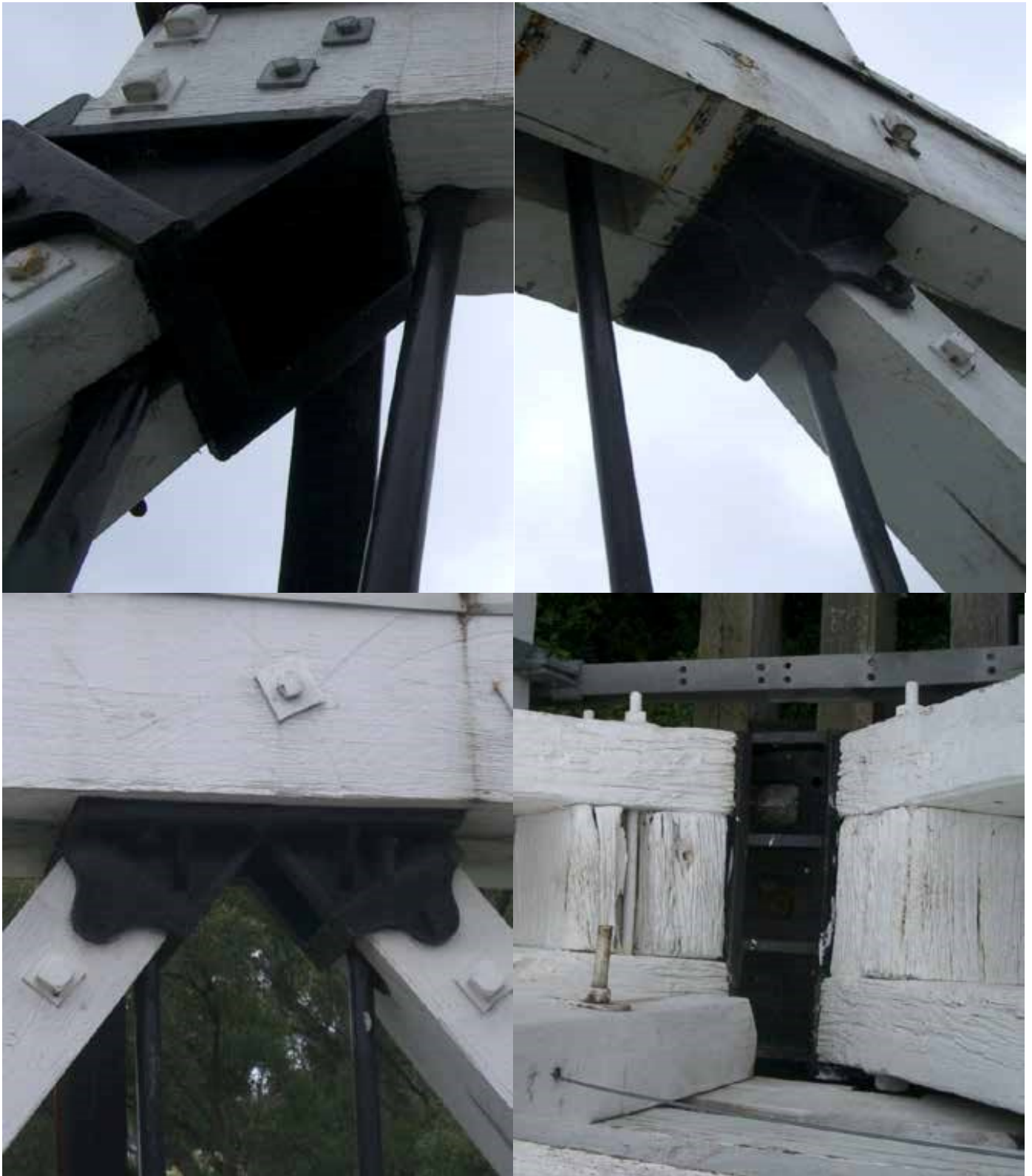
Figure 2-67: Photographs of various cast iron shoes at Victoria Bridge
