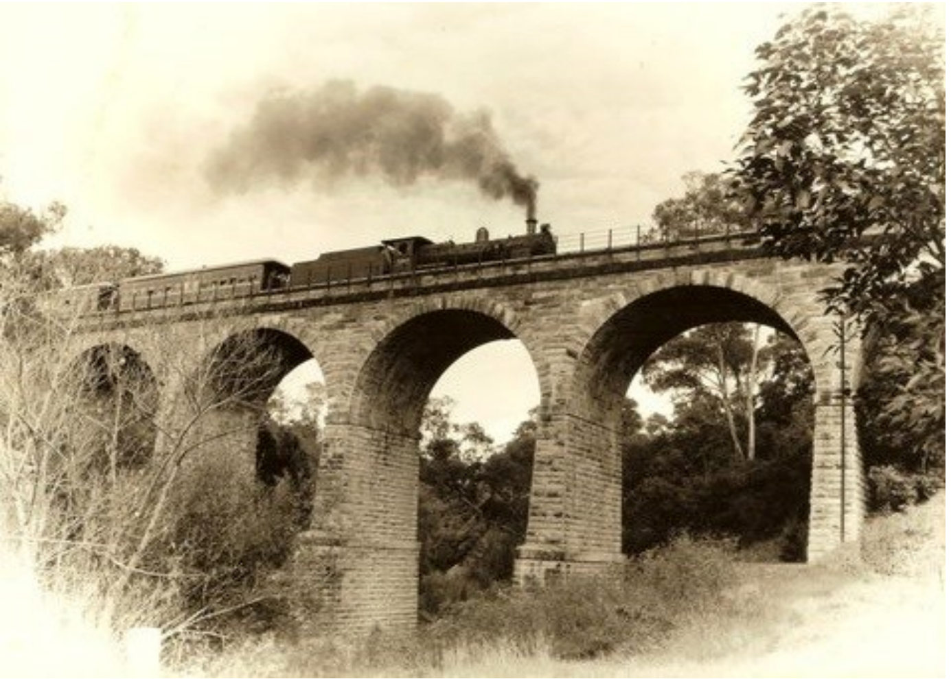
Figure 2-26: Railway Viaduct at Picton c. 1900
