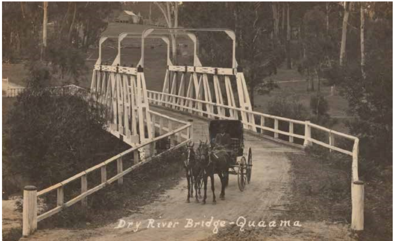
Figure 2-15: Early Allan truss with overhead bracing added, undated
