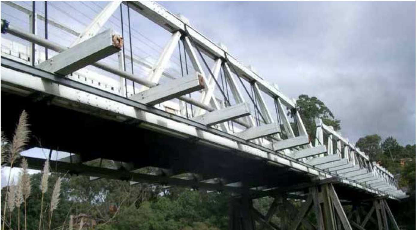
Figure 2-75: Maintenance monorail attached to underside of cross girders
