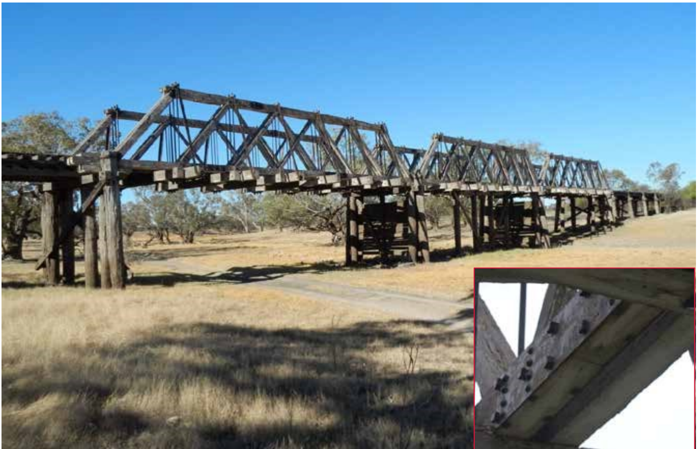
Figure 2-9: Rail bridge near Walgett NSW with Allan's bottom chord splice
