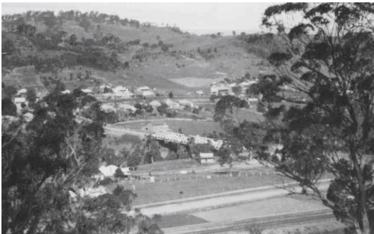
Figure 2-34: View of Picton looking east, 1920
