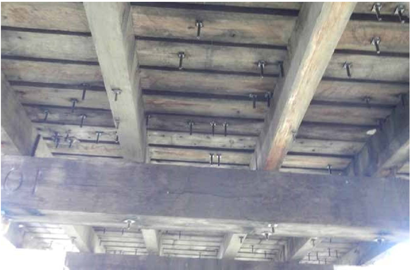
Figure 2-51: View of existing bolted deck from beneath Victoria Bridge
