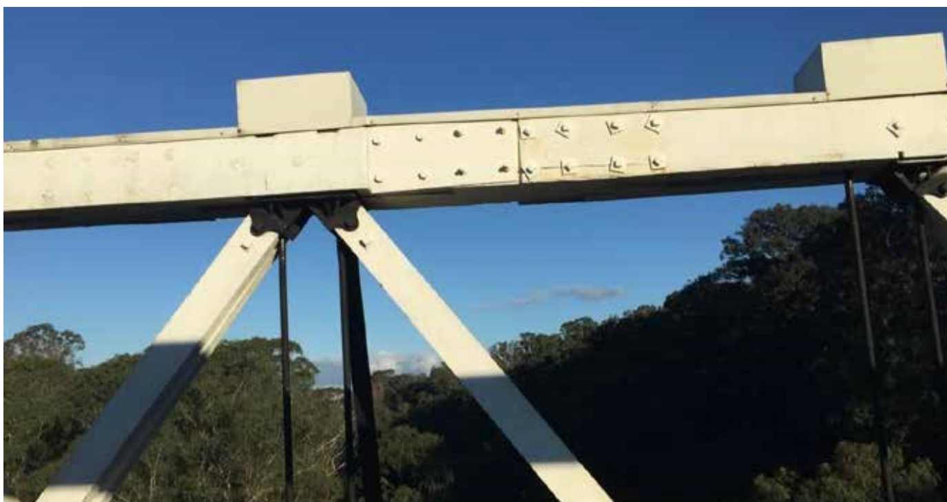
Figure 2-57: Additional splice at D-E in Span 2 Downstream
