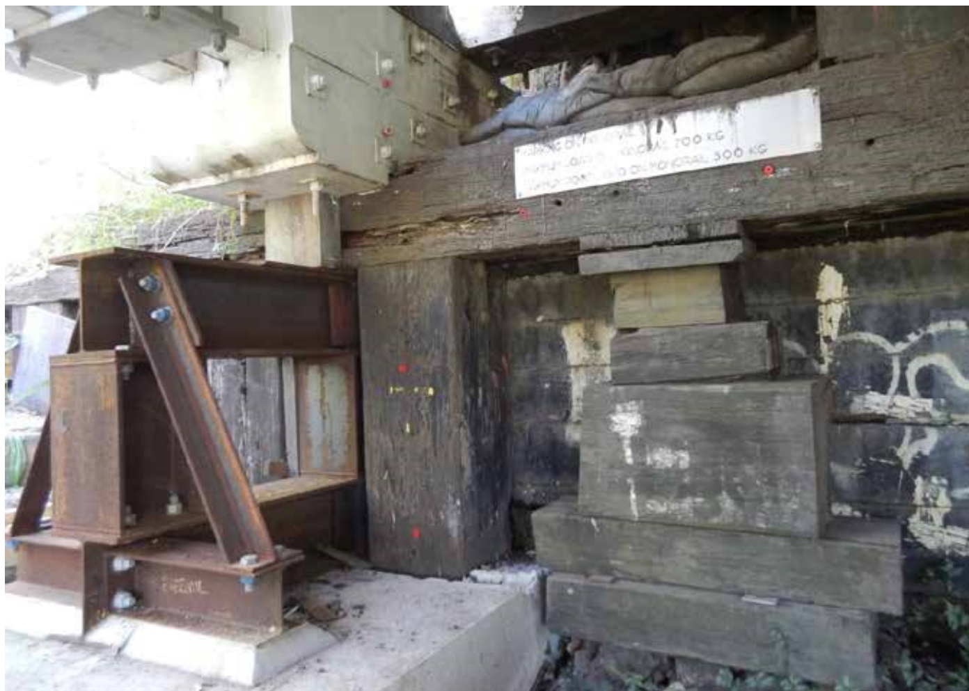
Figure 2-88: Photograph of Victoria Bridge Abutment A downstream side
