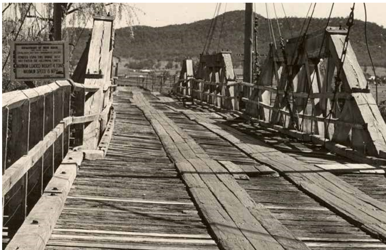
Figure 2-50: Typical Running Planks on Timber Bridge
