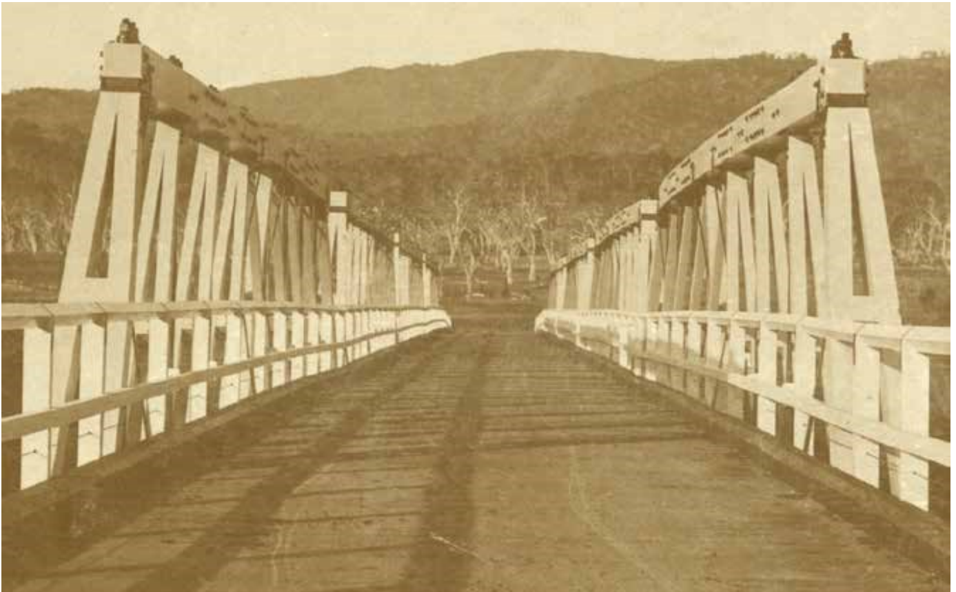
Figure 2-17: Original timber deck on Tharwa Bridge, undated
