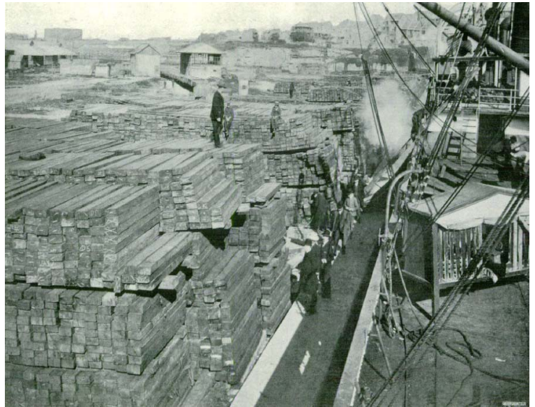
Figure 2.4: Australian Hardwood Sleepers and Girders being loaded at Darling Harbour for South Africa, 1903 17
