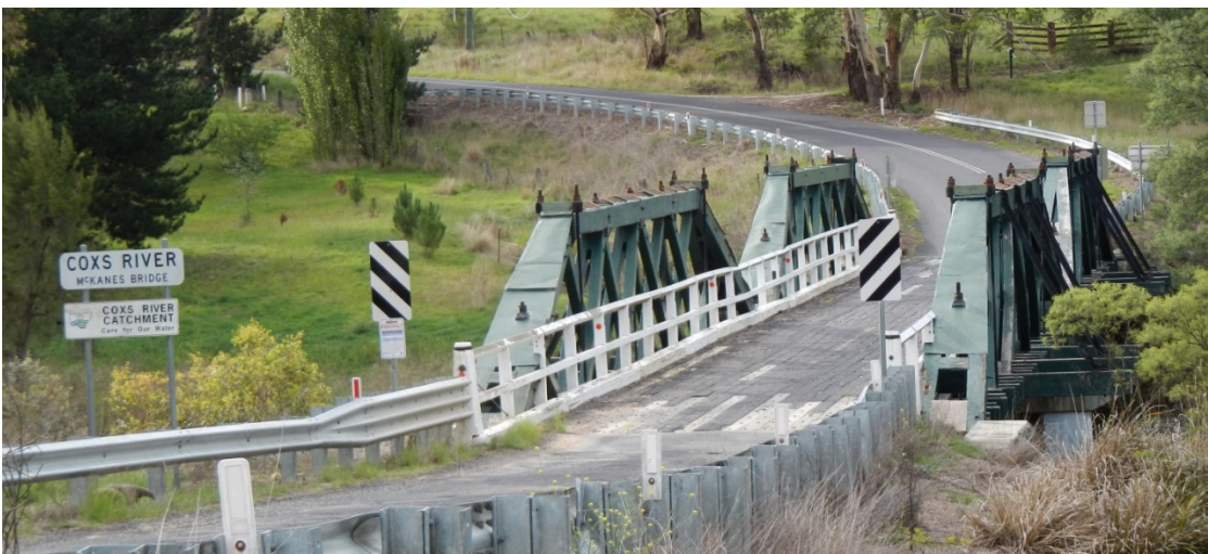
Figure 1-3: Photograph of McKanes Bridge in its setting from above.
