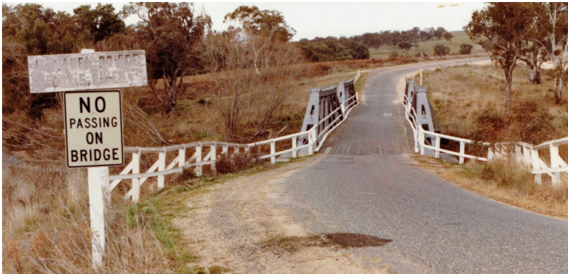
Figure 2-41: First colour photograph of bridge on file, taken 1979.
