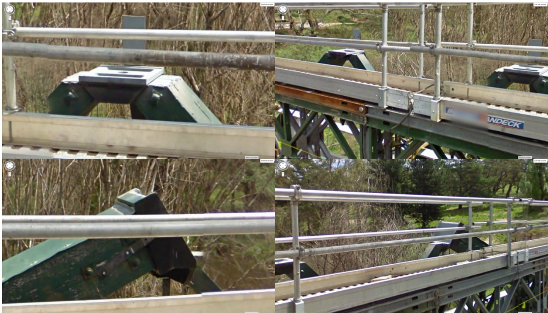
Figure 2-64: Top chord shoes of McKanes Bridge with top chord removed.
