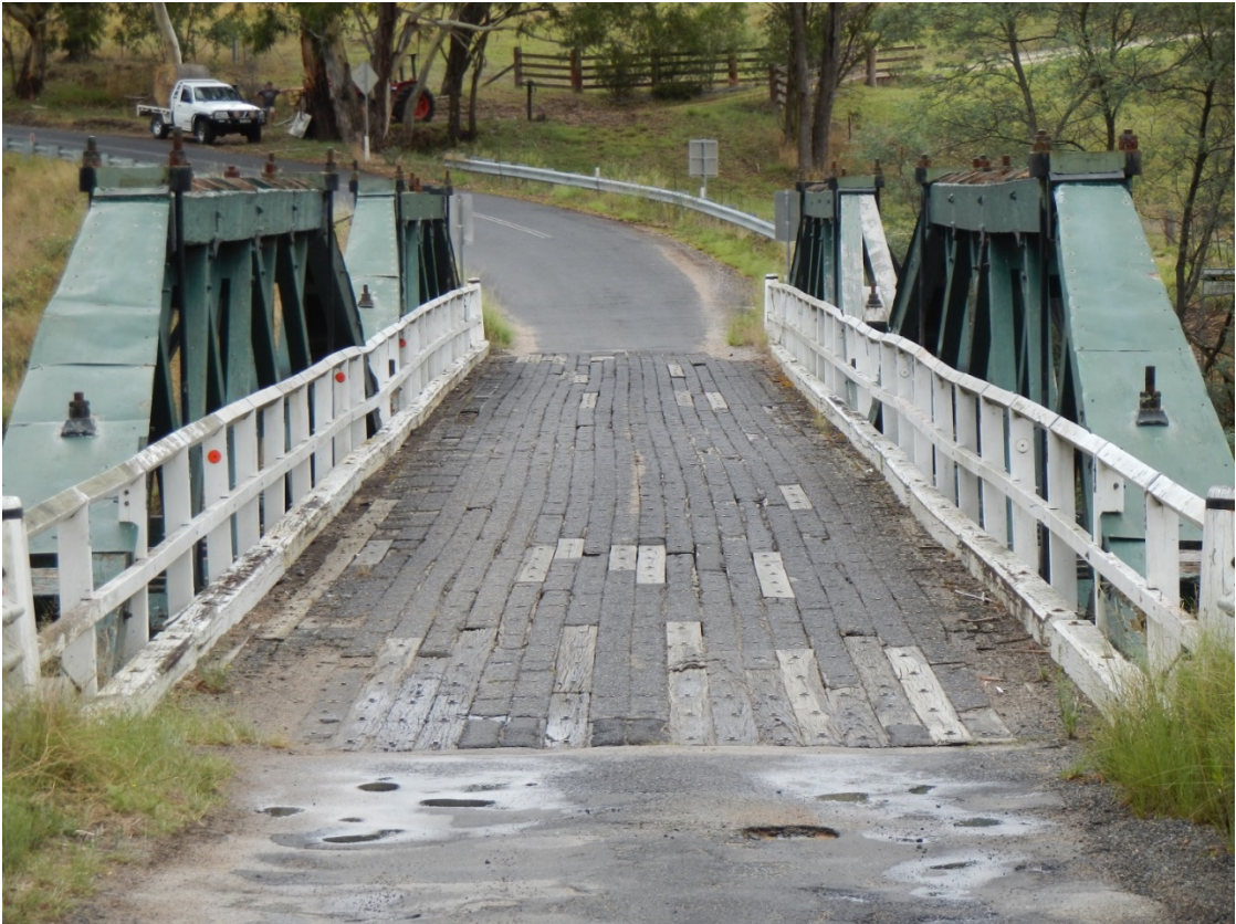
Figure 3-44: View of existing timber decking as seen from above.
