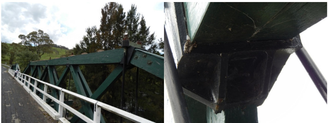
Figure 3-33: Photographs of typical cast iron shoulder shoe.
