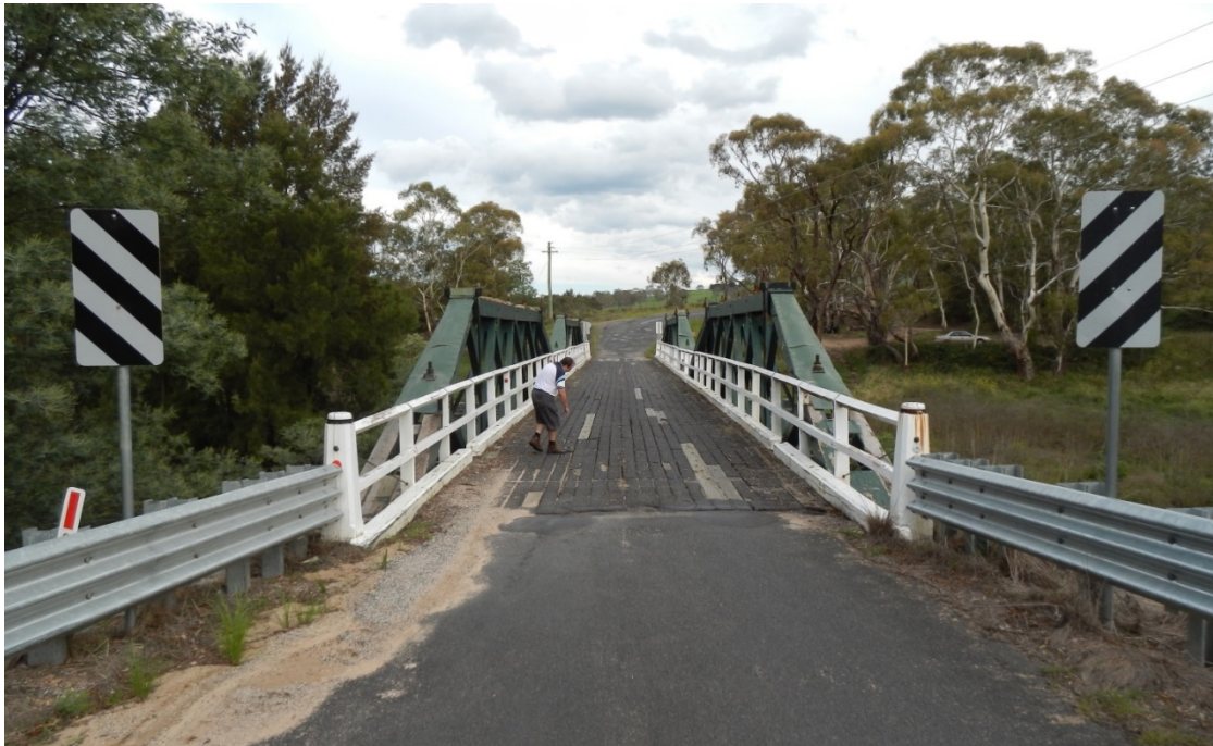
Figure 3-49: Photo showing new thrie beam guardrail on road approaches.
