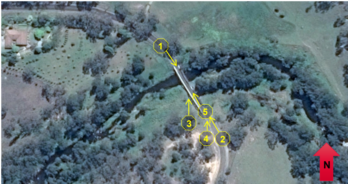
Figure 1-5: Aerial View of Bridge with locations from which views are seen.
