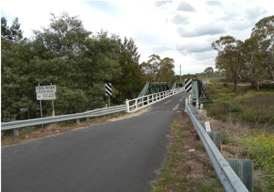
Figure 1-6: View 1 approaching the bridge from the north.
