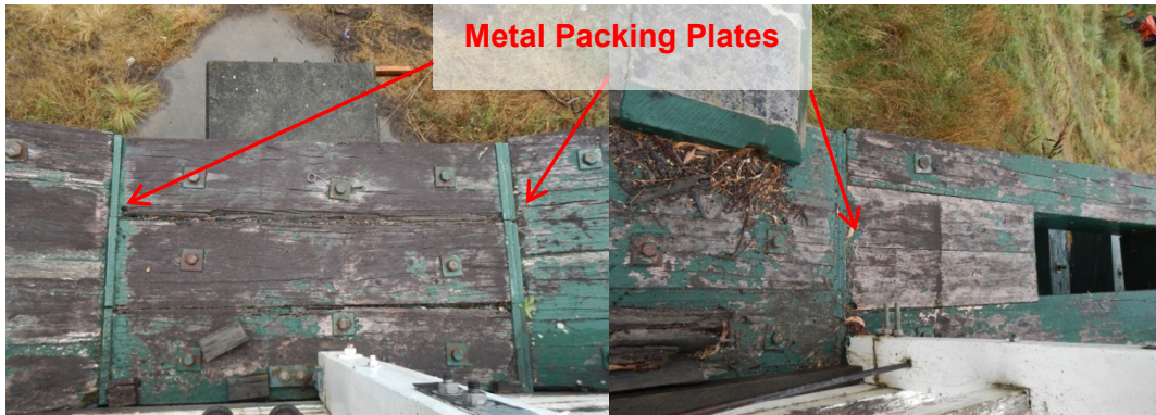
Figure 3-18: Metal packing plates introduced at the bases of principals.
