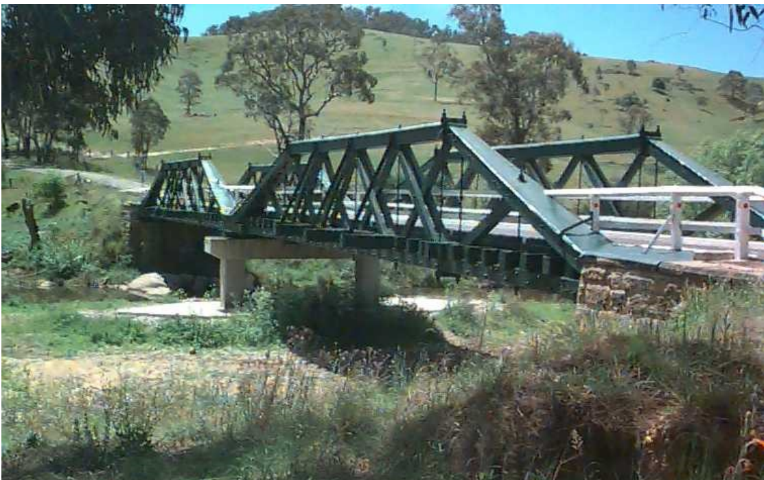
Figure 2-51: Photo showing concrete pier constructed in 1987.
