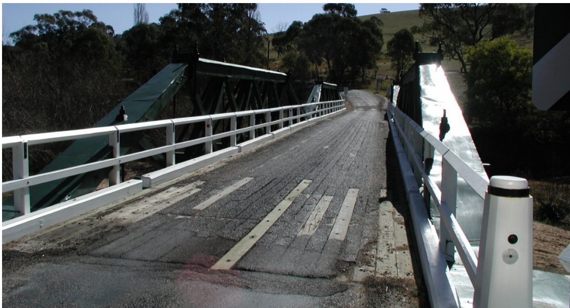
Figure 3-48: Photo of new railing installed after major works in 2001.
