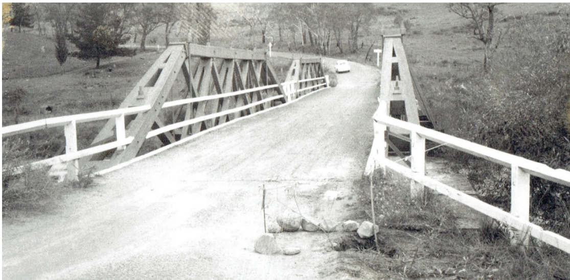
Figure 2-40: Bridge in 1978 with longitudinal timber sheeting.
