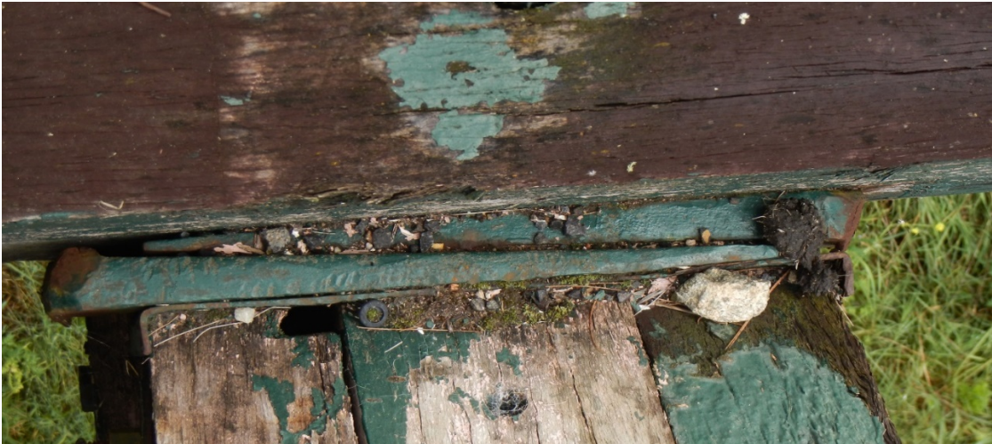
Figure 3-42: Photograph of typical metal wedges next to cross girders.
