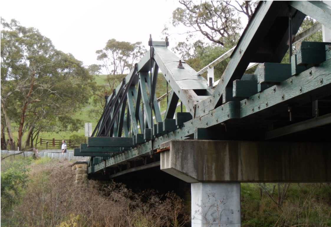
Figure 3-41: Photo of irregular and non-original lengths of all cross girders.
