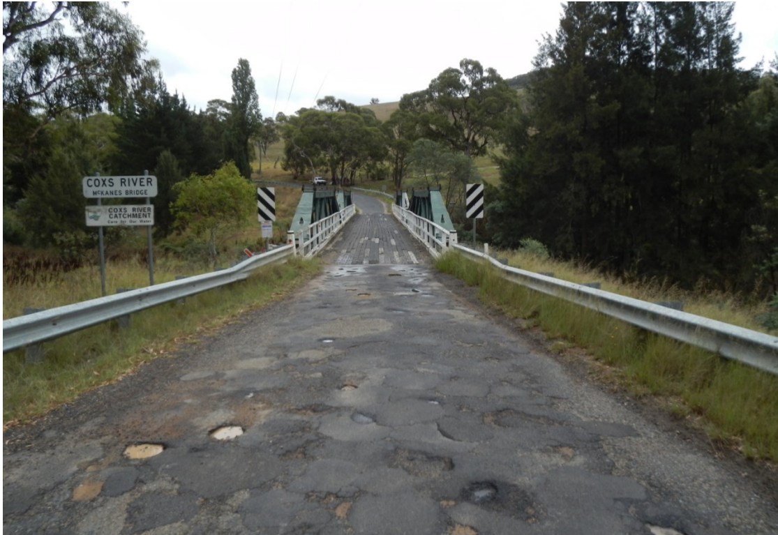
Figure 1-7: View 2 approaching the bridge from the south
