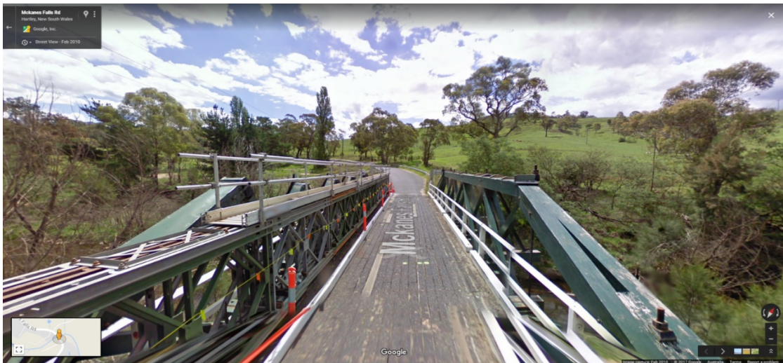
Figure 2-63: Google street view of McKanes Bridge in February 2010.
