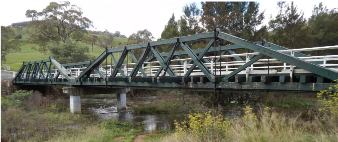
Figure 1-2: Photograph of McKanes Bridge in its setting from below.
