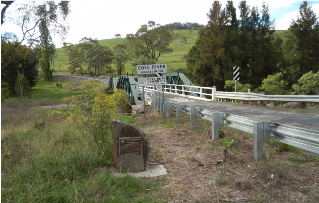
Figure 1-9: View 4 showing Engineers Australia plaque at southern end.
