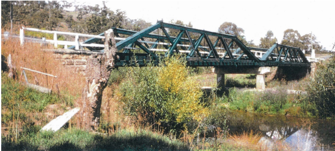
Figure 2-52: Photo showing bridge in January 1998.
