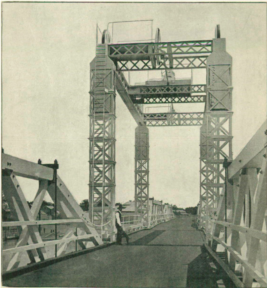
Figure 3-43: Original timber deck on McDonald truss bridge, Darling River at Wentworth, 1894. 103
