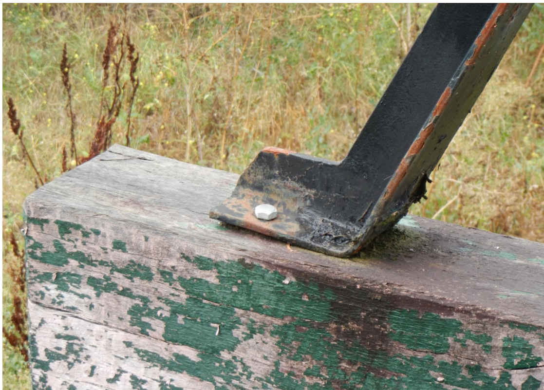
Figure 3-35: Photograph of base of typical sway brace at McKanes Bridge.
