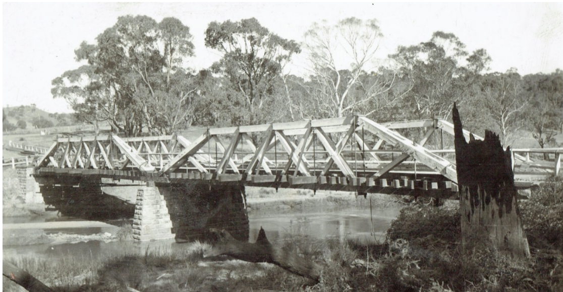
Figure 2-38: Earliest photograph found of McKanes Bridge in 1950.
