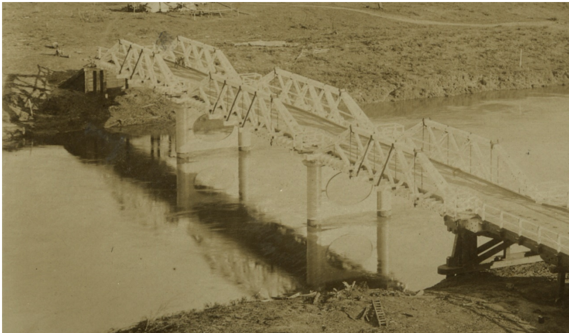
Figure 3-46: View of typical original McDonald truss.
