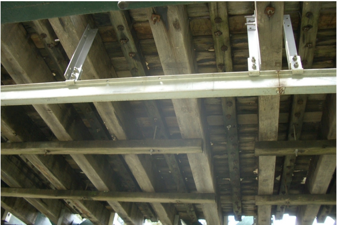
Figure 3-45: View of existing timber decking system as seen from below.
