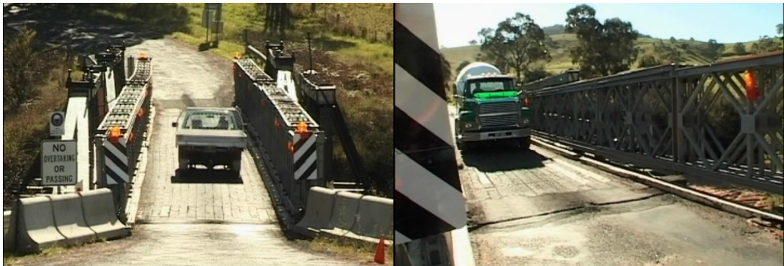
Figure 2-55: Timber trusses completely unloaded with Bailey trusses.
