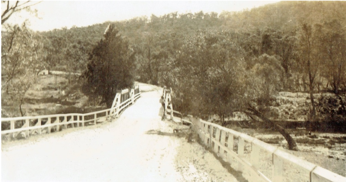
Figure 2-39: McKanes Bridge in 1954.
