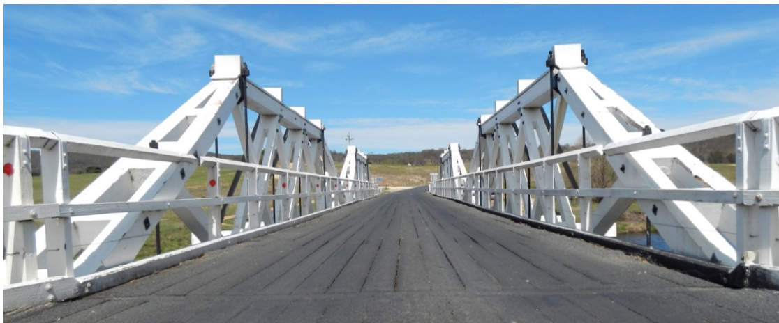
Figure 2-14: Splayed principals of McDonald truss, Bombala.
