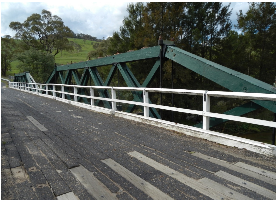
Figure 3-2: Photo of top chords with packers on top for metal flashing.
