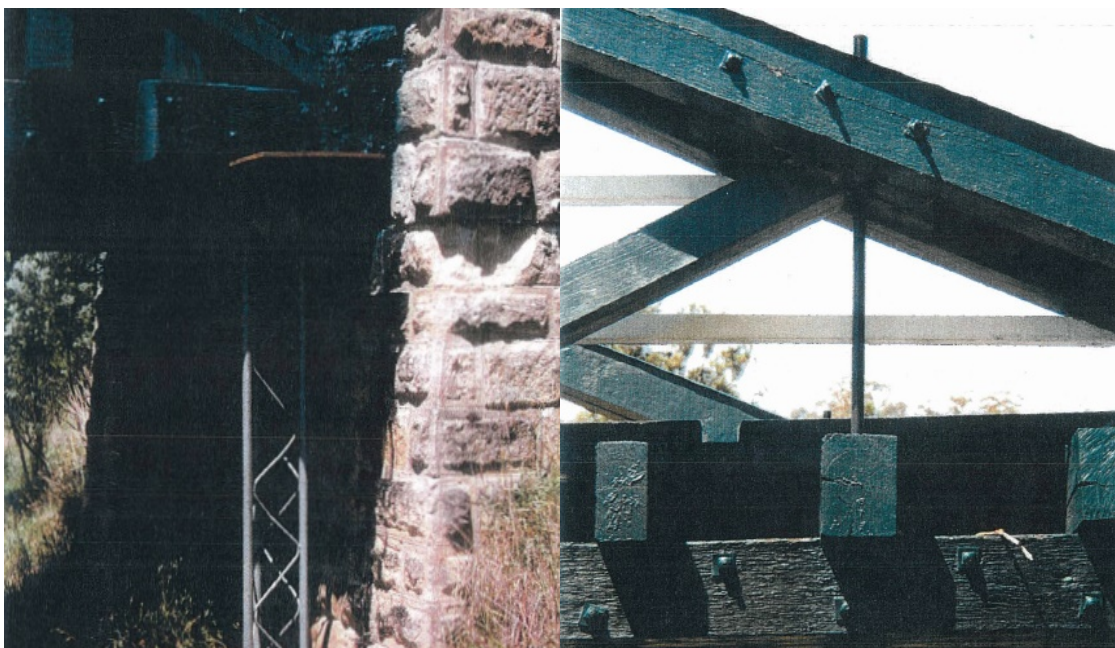
Figure 2-53: Photo of loose members and Tri-shore.
