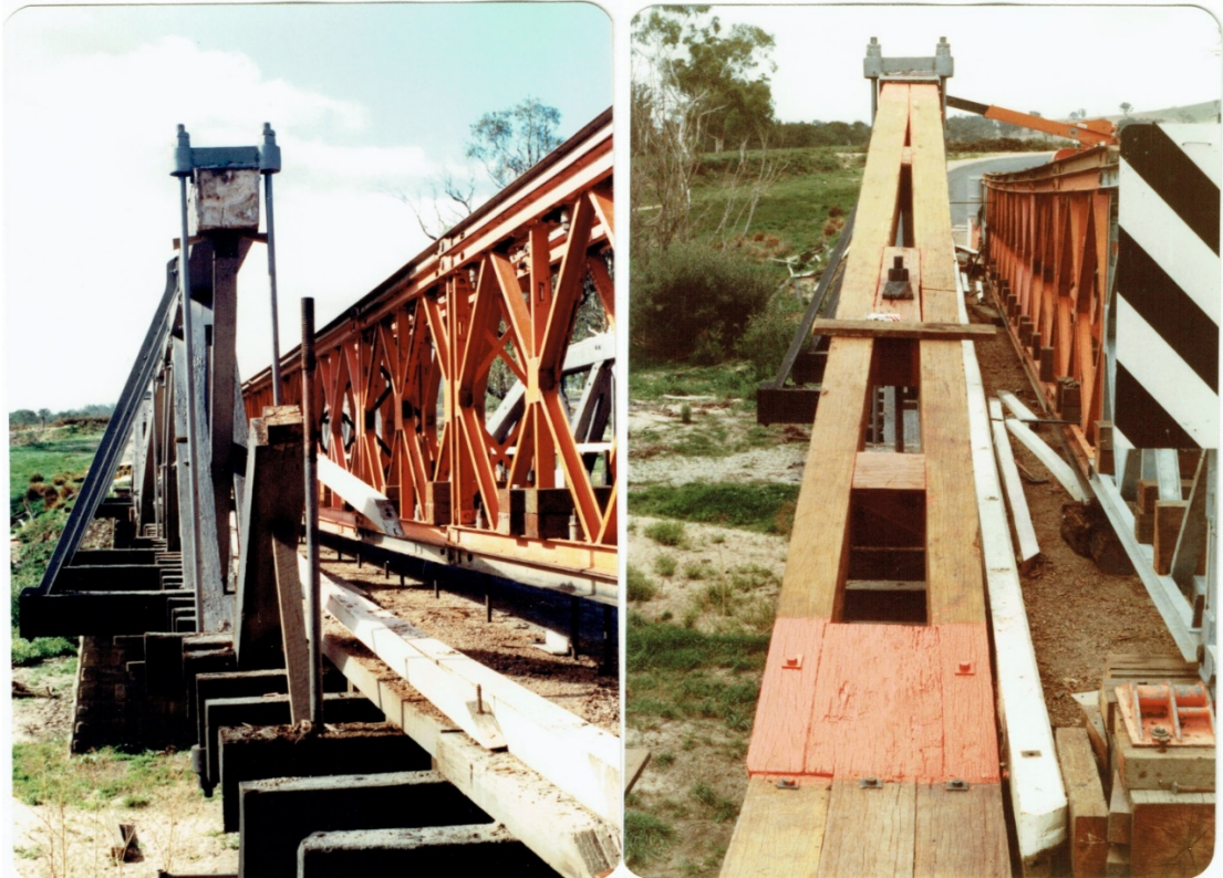
Figure 2-43: Photographs showing replacement of principal, 1982.
