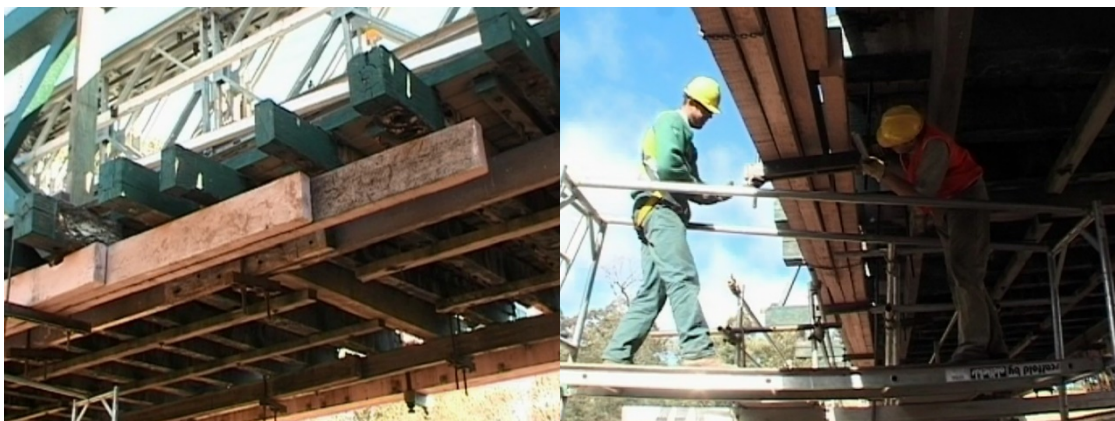
Figure 2-58: Replacement of laminated timber bottom chords.
