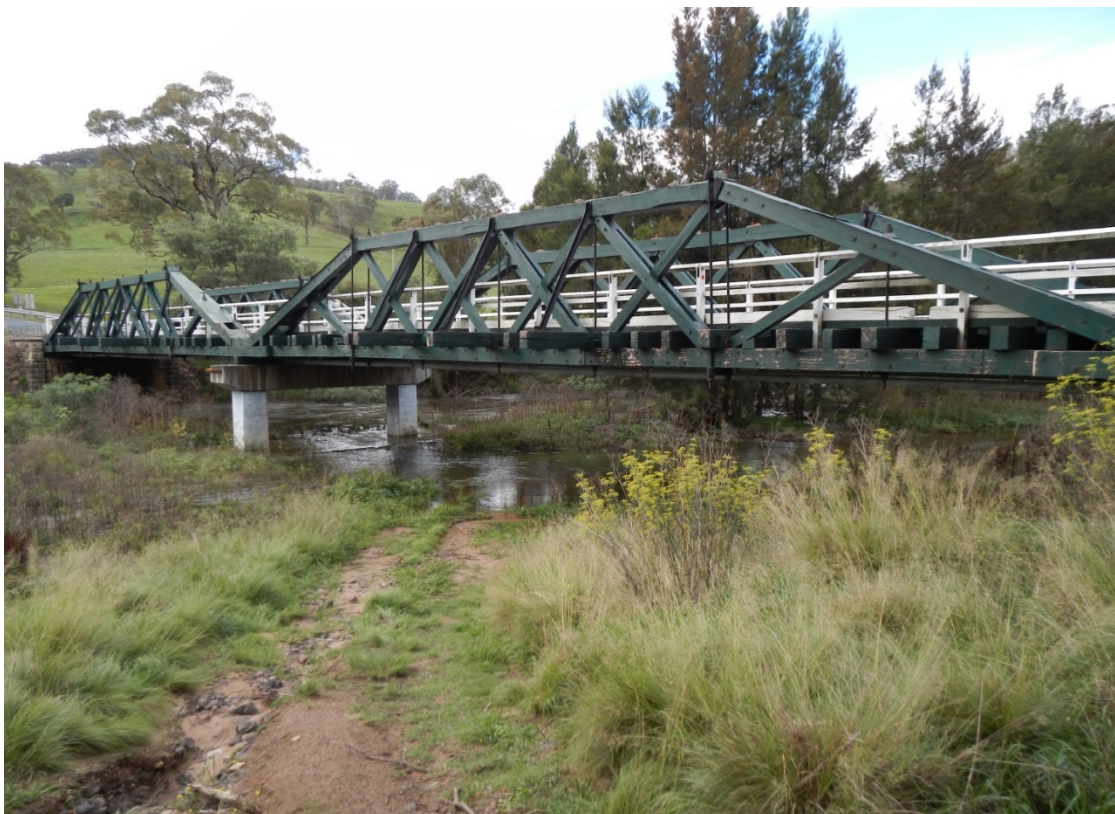
Figure 1-8: View 3 from southwestern side of the bridge.
