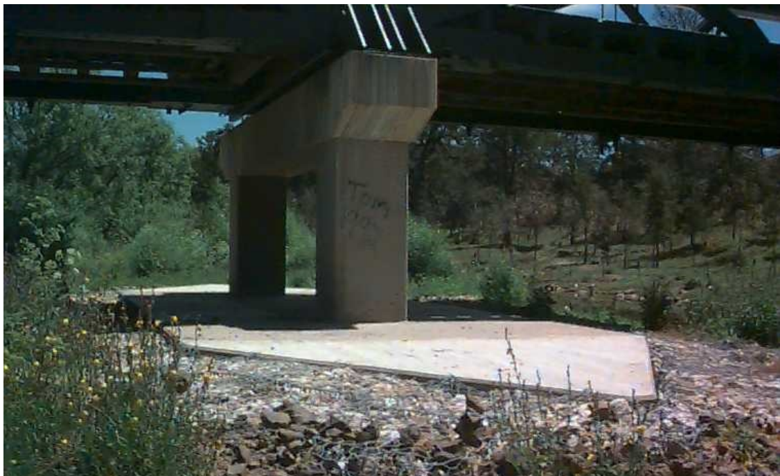
Figure 3-53: Photo of new pier taken between 1987 and 1999.
