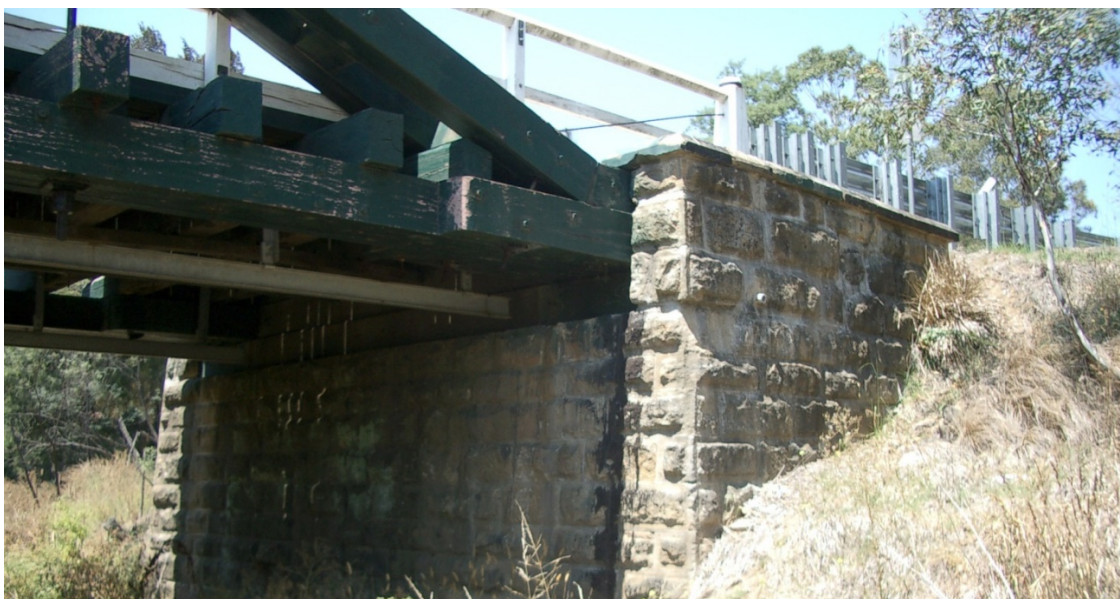
Figure 3-51: Photograph of masonry abutment largely as original.
