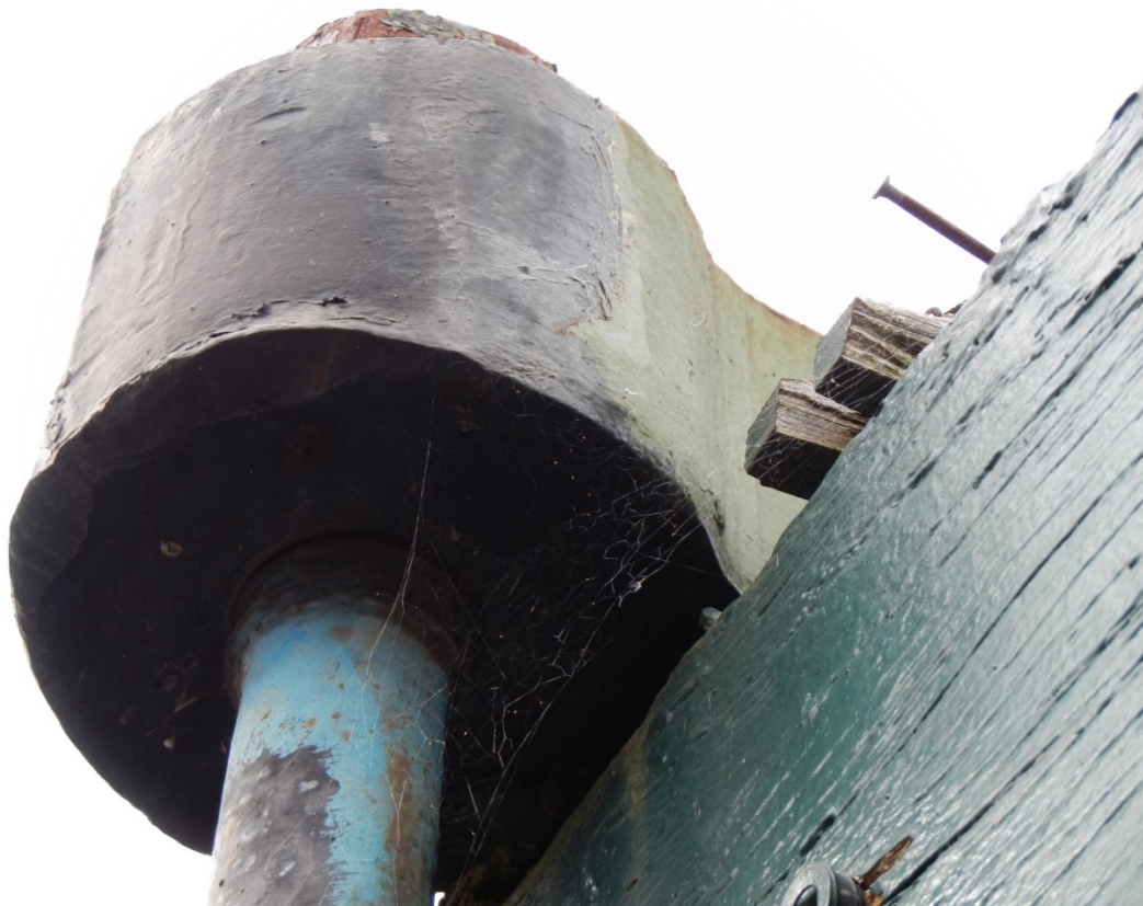
Figure 3-26: Photograph top of tension rod showing upsized threaded end.
