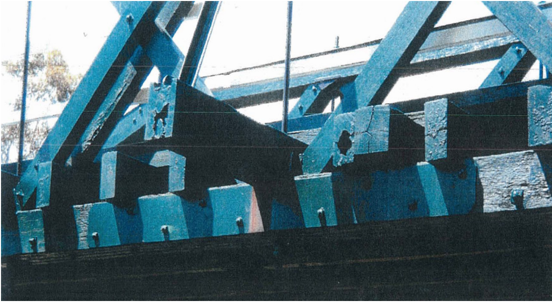
Figure 3-9: Comparison of bottom chord in 1998 (above) and 2013 (below) with no splice plate. 100
