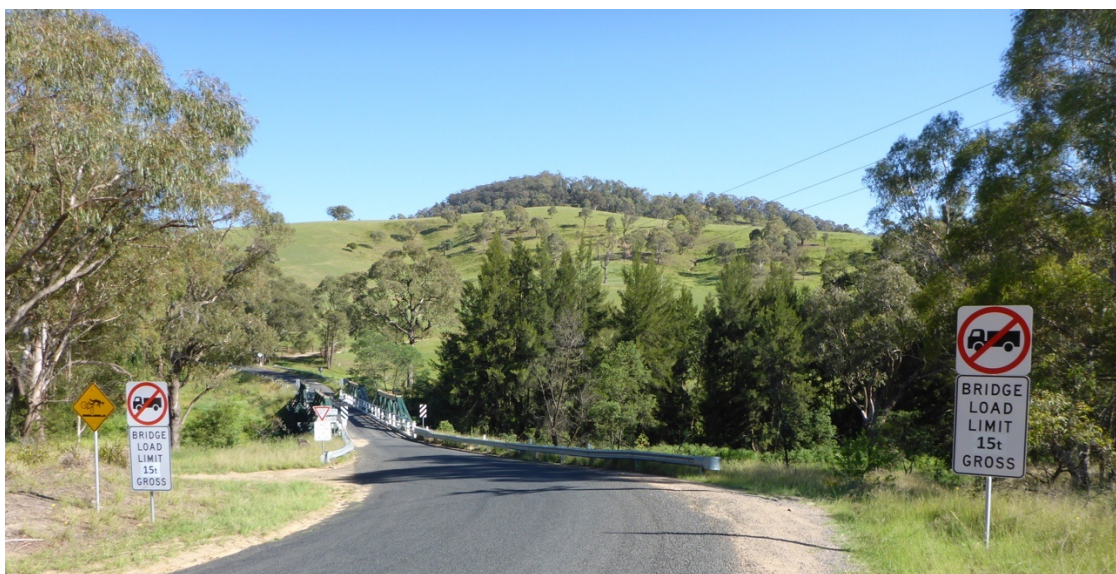
Figure 2-65: Load limit and warning signs at bridge approaches.
