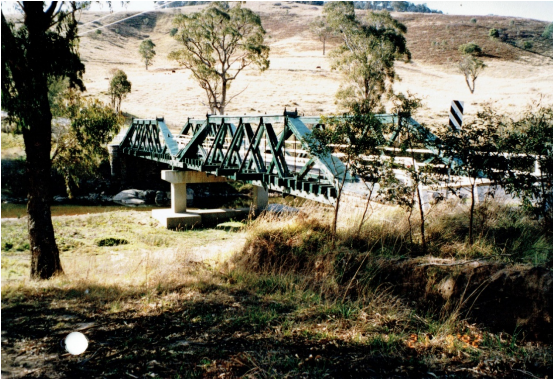
Figure 2-50: 1992 photo of concrete pier as constructed in 1987.
