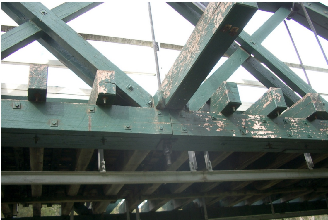
Figure 3-37: View of larger primary and smaller secondary cross girders.
