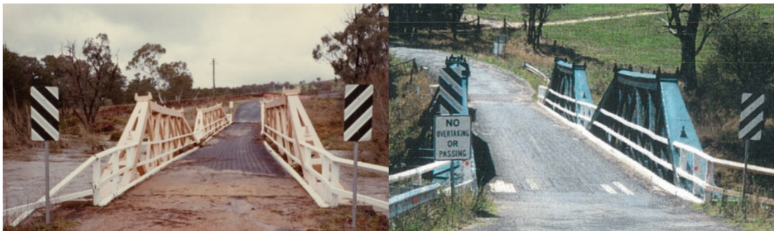
Figure 3-47: Photos showing railing against different truss colours in 1986 (left) and 1998 (right). 107
