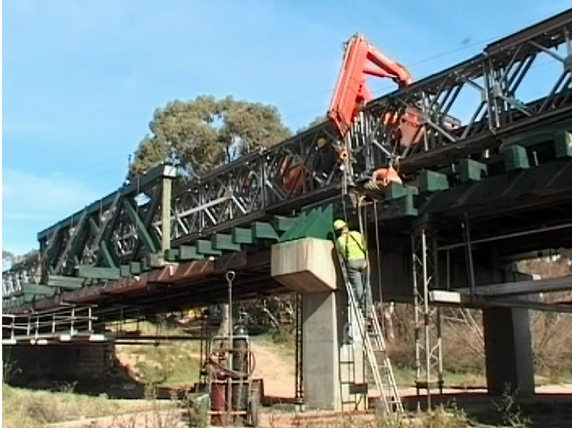
Figure 2-57: Disassembly of bridge to replace bottom chords.
